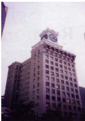
Figure 4: The north and west elevations of the Vancouver Block Building after the rehabilitation works.
