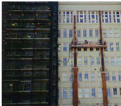
Figure 2: The use of swing stages and scaffolding during the rehabilitation works.
