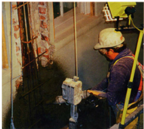
Figure 3: The application of shotcrete from a swing stage.
