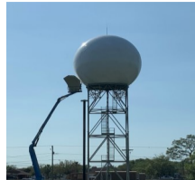
KTBW Radar Dome Replaced
