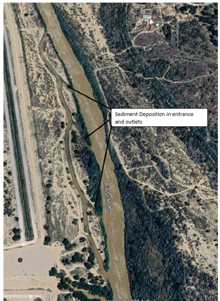
Constructed side channel after several years of inundation during spring runoff and monsoon thunderstorms.
