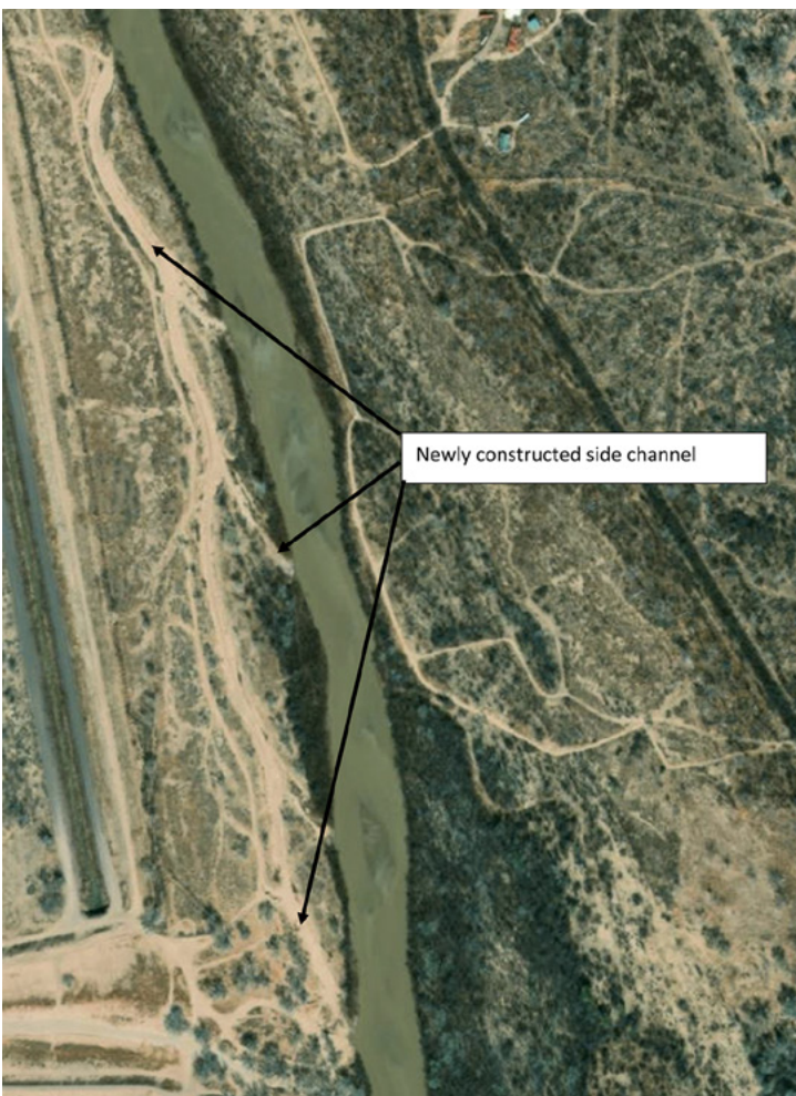
Newly constructed habitat features that includes several connections to the main channel.
