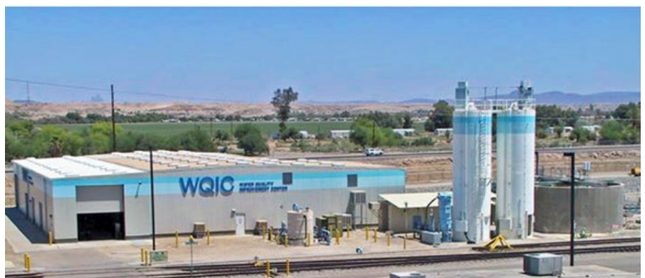
Reclamation's Water Quality Improvement Center in Yuma, Arizona.
