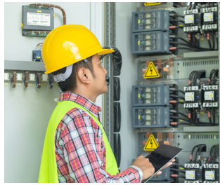
Safe Power Limit
