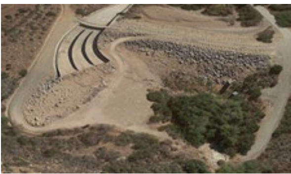
g. Post-fire accelerated sedimentation rates in Santa Monica Debris Basin in Carpinteria, CA. The 208,000 yd 3 capacity basin (approximately 100 ft deep) (left photograph) was almost completely filled with sediment after a single storm on Jan. 9, 2018. Rain fell at a rate of 1 in/hour over a burnt watershed area (3.8 mi 2 ) and produced an influx of over 150,000 yd 3 of sediment within 1 hour. The sediment production rate of 40,000 yd 3 /mi 2 after wildfire is not unusual. Rates exceeding 130,000 yd 3 /mi 2 have been documented in a single storm in these fire-flood situations. Such events often require intensive emergency sediment removal to restore capacity before additional storms occur. This is a good example of how increased incidence of wildfire can increase sediment yield. Extensive drought (perhaps associated with climate change) can increase the occurrence and severity of wildfire.
