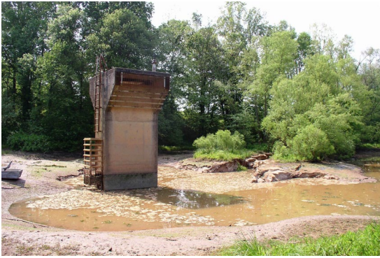
e. Reservoir sedimentation is beginning to bury the outlet works at Deep Creek Dam, NC, 2007.
