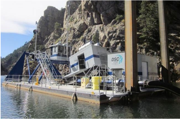
p. Hydraulic dredging of sediments from Strontia Springs Reservoir, near Denver, CO, for transport through a sediment slurry pipeline to downstream areas of Waterton Canyon. Accelerated post-fire sedimentation impacted water quality. Wood and sedimentation have affected the dam outlet (Raitt and Cochran, 2017).
