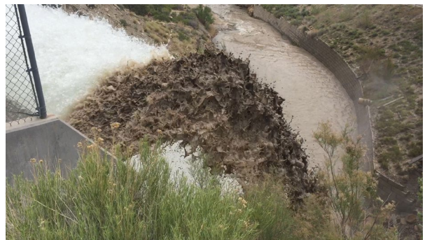
s. Sediment releases down the spillway of Millsite Dam near Ferron, UT (photograph courtesy of Rollin Hotchkiss).
