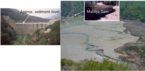
j. Sedimentation has almost completely filled the reservoir behind Matilija Dam near Ventura, CA.
