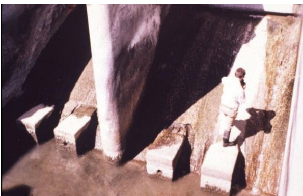
n. Sand has abraded the spillway at the Milburn Diversion Dam near Sargent, NE.
