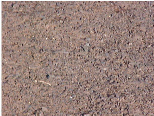
Figure 4. Close-up of Walkway Made from Waste Tire Chips
