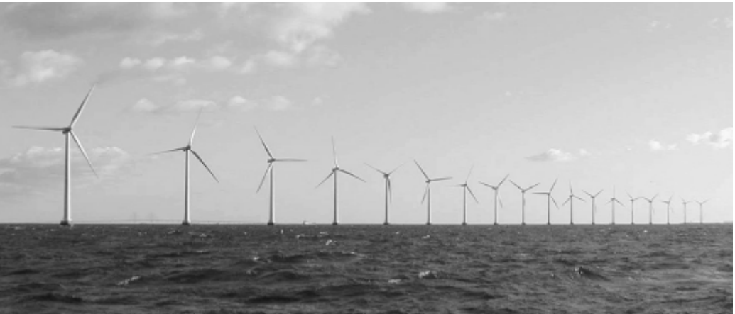
Figure 11.4 The Middelgrunden wind farm. Photo by Jens H. Larsen and Mads Eskesen. Published with the permission of Københavns Miljø og Energikontor
