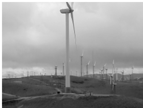
Figure 23.6 Enron Wind 1.5-MW turbine located near Tehachapi, California
