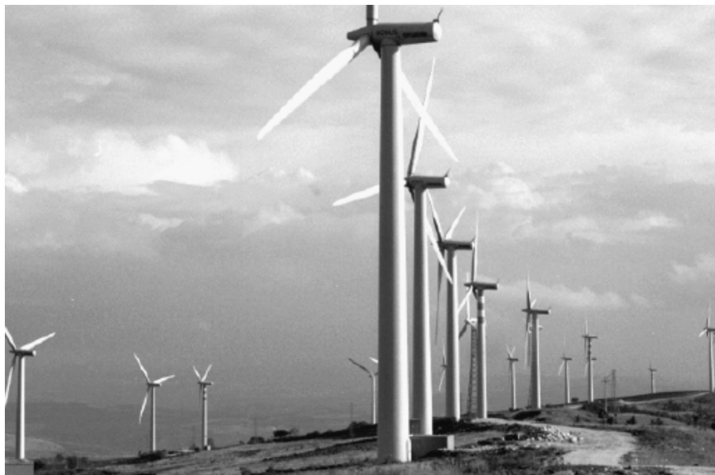
Figure 15.6 Filippo Sanseverino windfarm at Castelfranco in Miscano (2 wind turbines Vestas 600 kW and 48 Bonus 600 kW)
