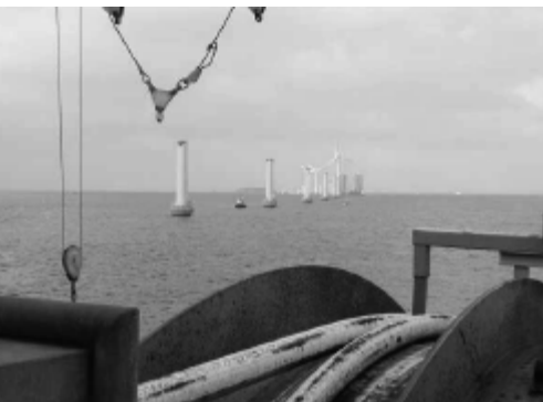
Figure 11.5 The Middelgrunden wind farm under construction. Photo by Jens H. Larsen and Mads Eskesen. Published with the permission of Københavns Miljø og Energikontor
