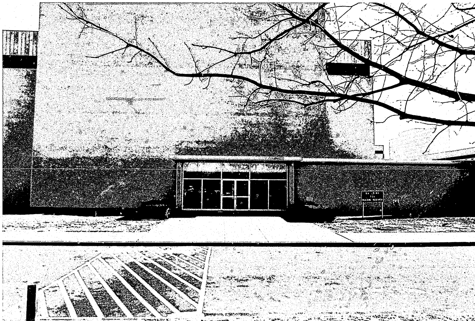
FIGURE 2. WEST FACADE OF A TYPICAL GPL BUILDING AT NBS GAITHERSBURG.
