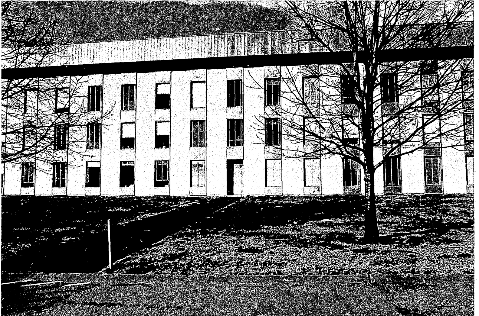
FIGURE 8. BLIND POSITIONS ON A TYPICAL NBS BUILDING FACADE.
