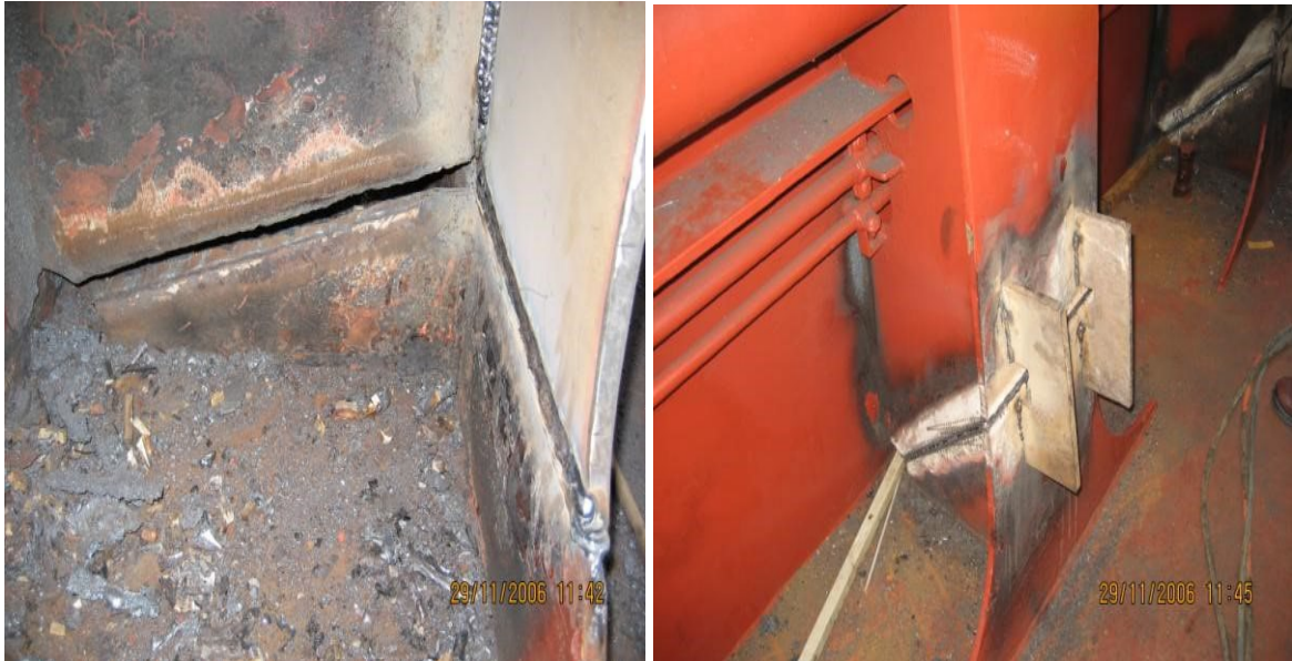
Figure 4 Return hatch coamings by cutting and welding of coamings stool [5]
