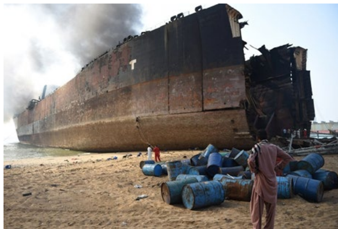
Figure 1 Gadani Shipbreaking site, Pakistan
