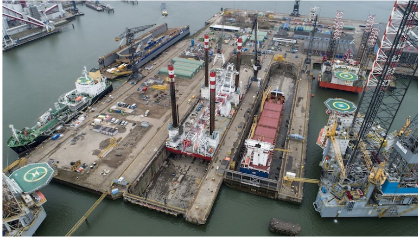
Figure 6 EU compatible recycling plant in the UK
