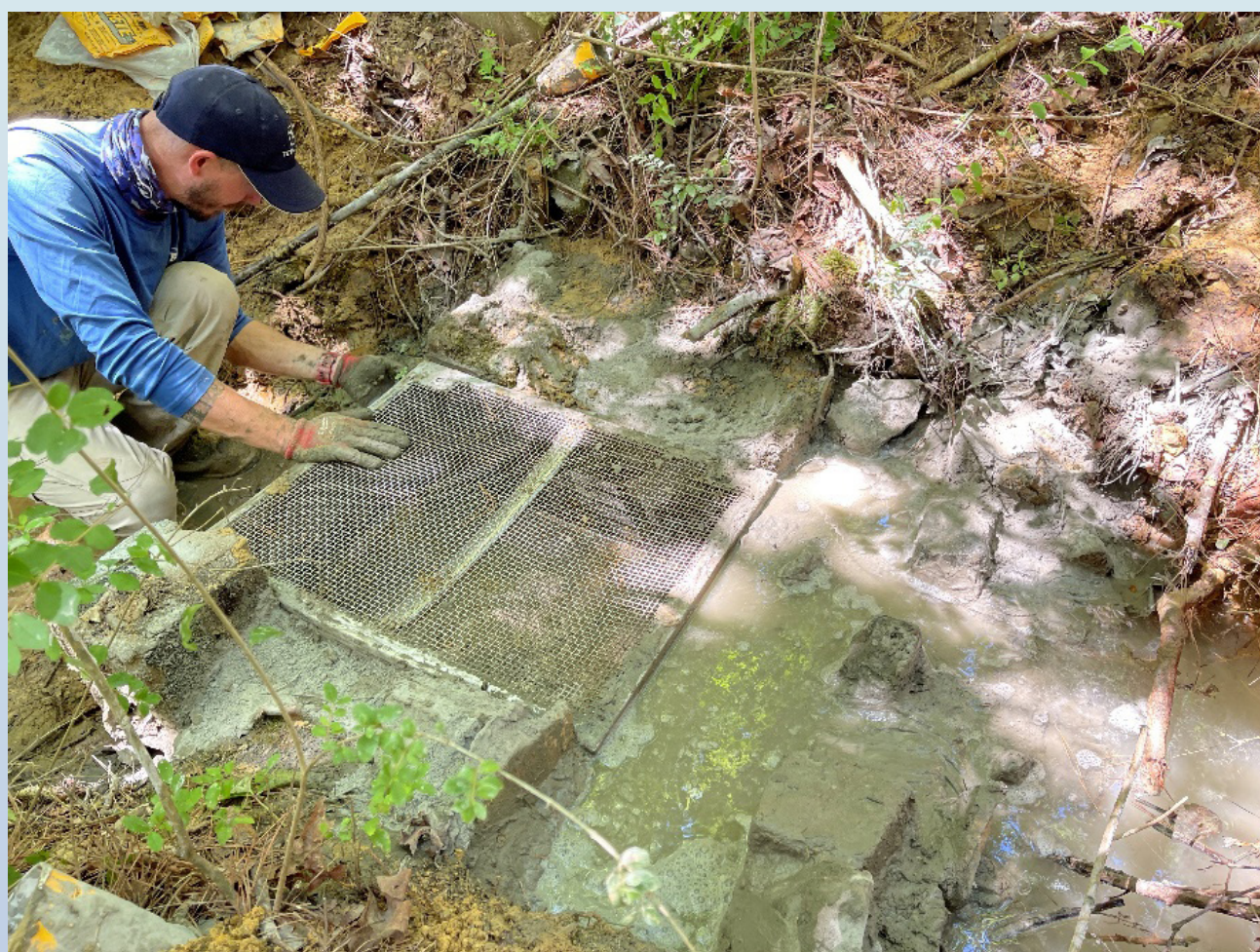
NASA designed a treatment system to remove PFAS from surface water near Outfall 3.
