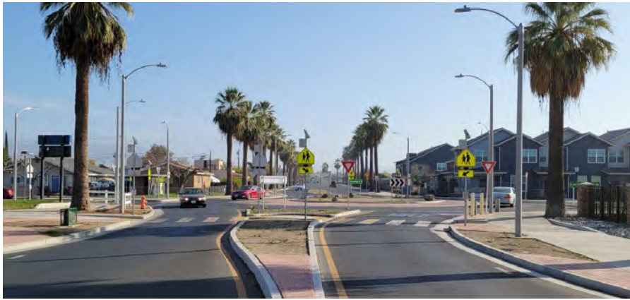
Roundabout at Westwood Avenue
