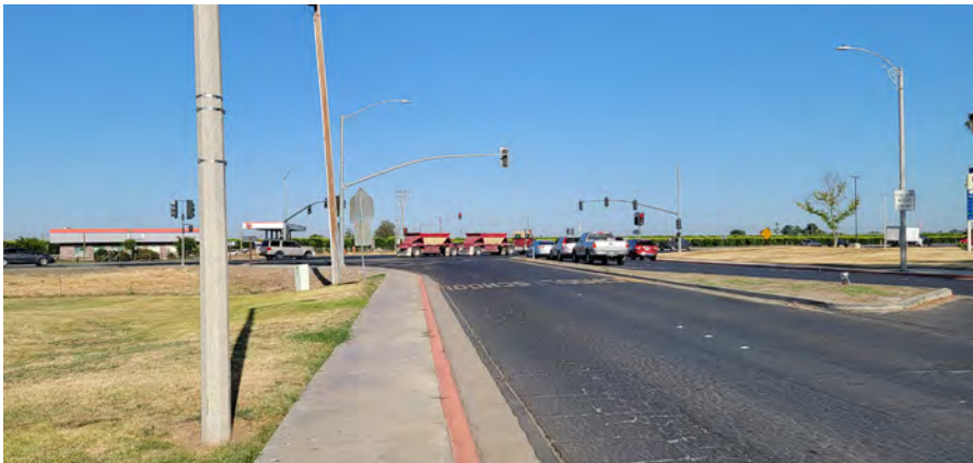
Existing sidewalk near State Route 65, lack of parkway
