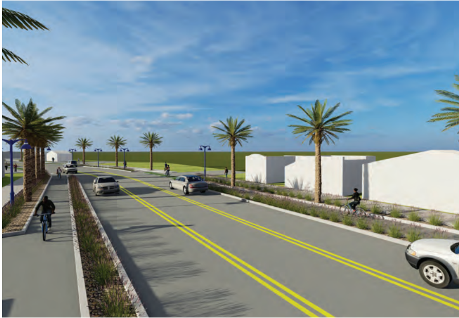
Proposed Class IV separated bikeway, center turn lane, and pedestrian enhancements such as lighting; looking west
