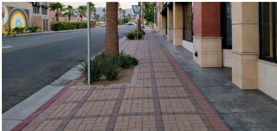
Enhanced sidewalks; paving patterns
