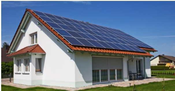
Figure 1. Solar panel on building roof, example of an active solar - PV system (Berkeley Lab, 2010).
