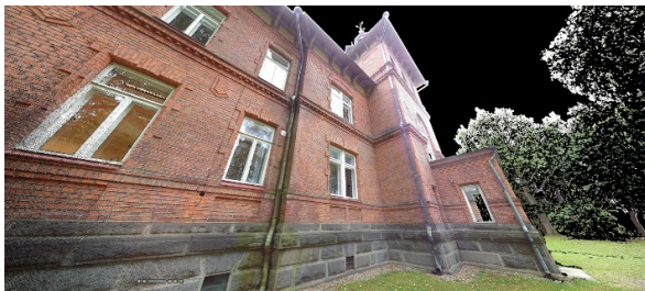
Figure. 1. Outdoor scan station and point cloud data obtained in the Lielahiti mansion campaign, 2016
