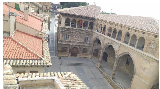
Figure 1. Exterior from the Town Hall of Alcañiz (Teruel)
