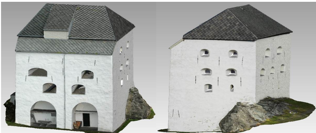
Figure 3: Perspective view of the defence tower (Donjon) modelled from point clouds – manual texture mapping on meshes in Geomagic
