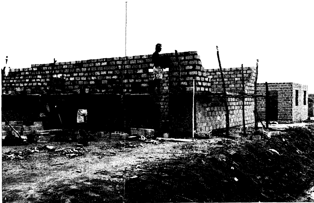
Construction of housing by family members involved in the Land Reform and Poverty Alleviation Pilot Project.
