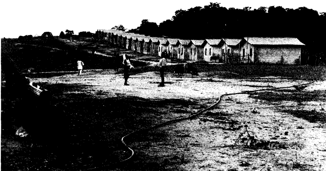
Partially completed houses at a Project site.
