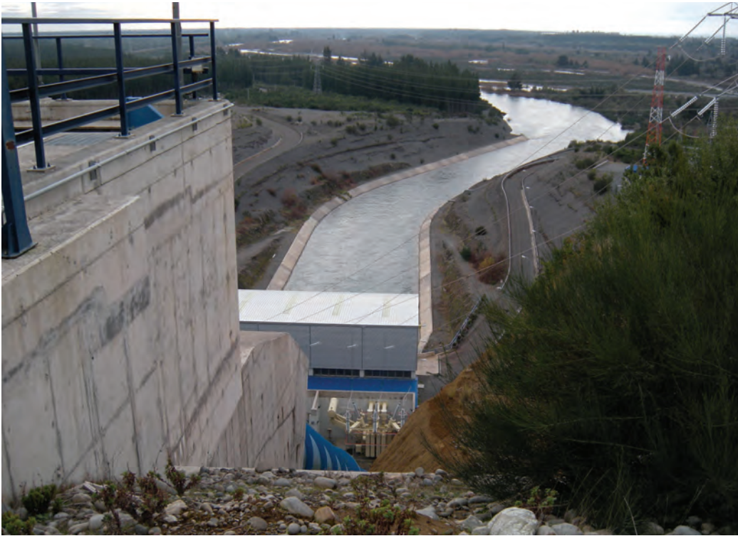
Chile: Quilleco Hydropower Project
