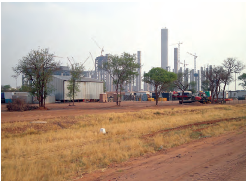
South Africa: Eskom Investment Support Project—site of Medupi Power Plant
