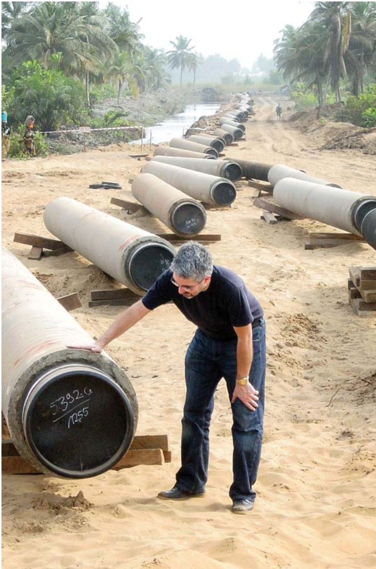
Inspection Panel at the right of way (ROW)
