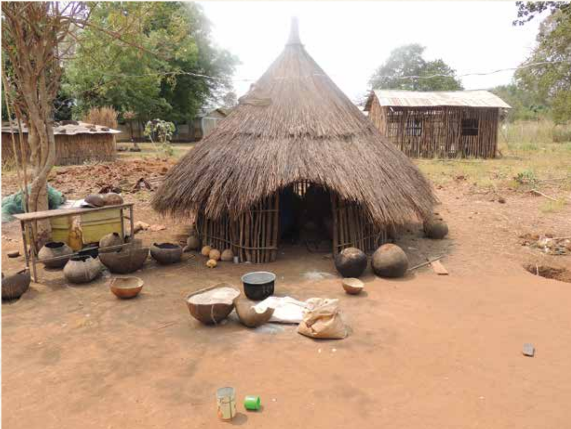
A hut in a community in Gambella, Ethiopia: Promoting Basic Services Phase III Project.
