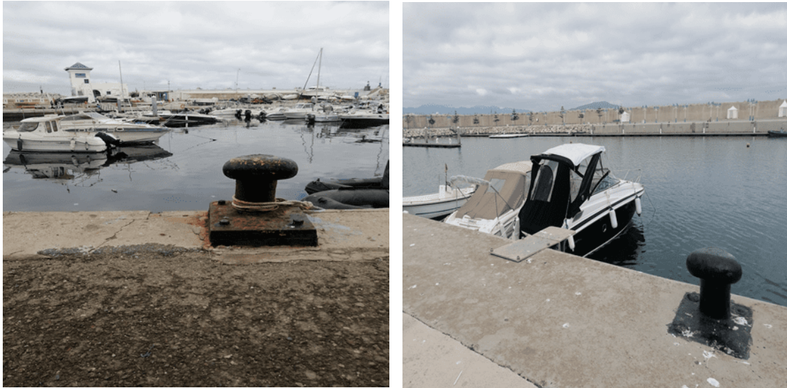
Fig.1. Images of a real-world A60 steel bollard case in port infrastructure.
