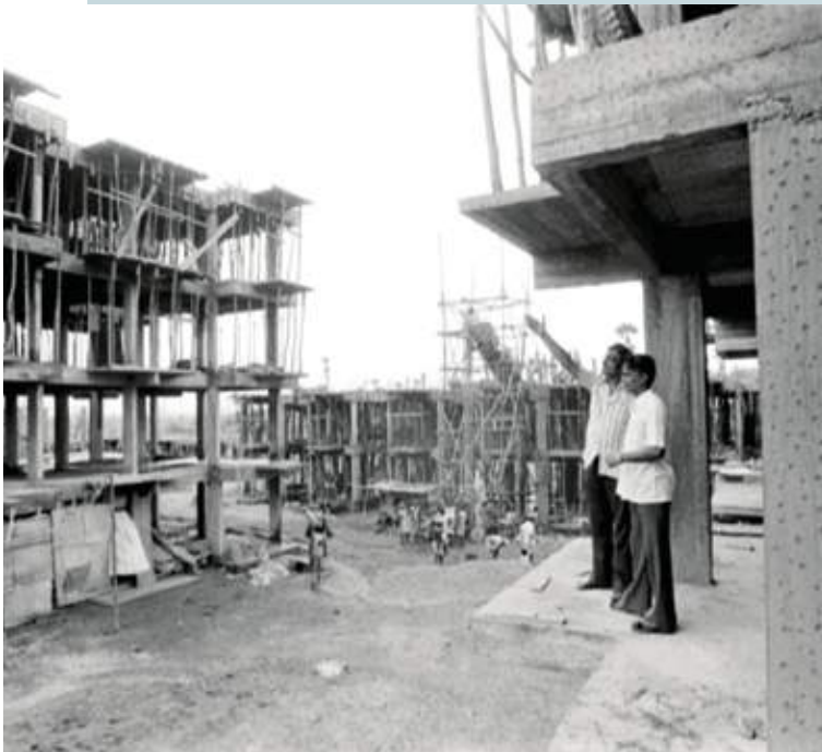
India: HDFC-financed housing units under construction, 1980.
