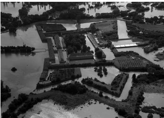
Fig. 7 Terezín, fortress. The original fortifications are based on Baroque fortification systems of the 17th century. During the August 2002 floods, Terezín and surroundings were flooded up to a height of 3 meters. The historically valuable underground protection system of the fortress was also badly damaged.
