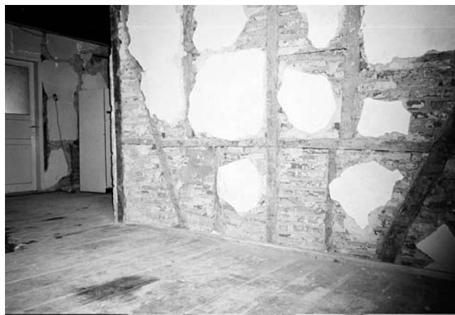
Fig. 12 Hımış interior wall in a house in the Düzce earthquake damage district showing »working« of wall that caused loss of plaster (photograph © Randolph Langenbach)
