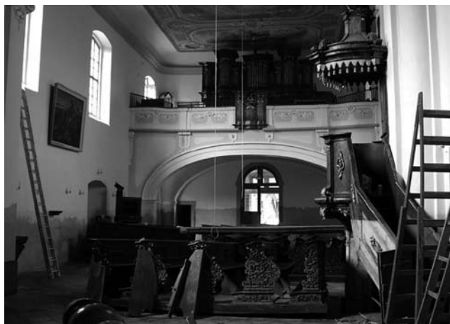
Fig. 10 Štětí, area of St. Simon and Juda Church, 1785. Church foundations at the sidewall were undermined; plasterwork, stone components and movable objects are damaged.
