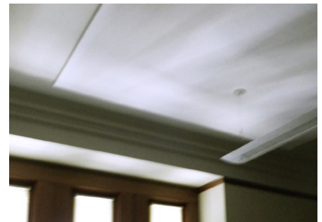
AFTER: Stretched acoustic material applied to ceiling
