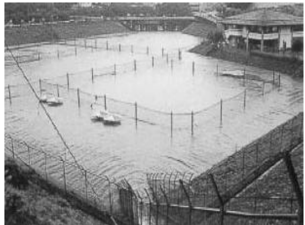
Figure 12: Multipurpose detention basin in Japan
