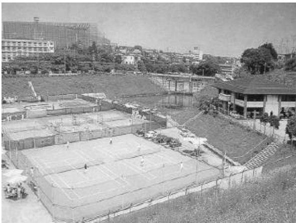
Figure 12: Multipurpose detention basin in Japan
