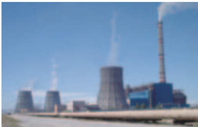
Ulaanbaatar Thermal Power Plant No.4
