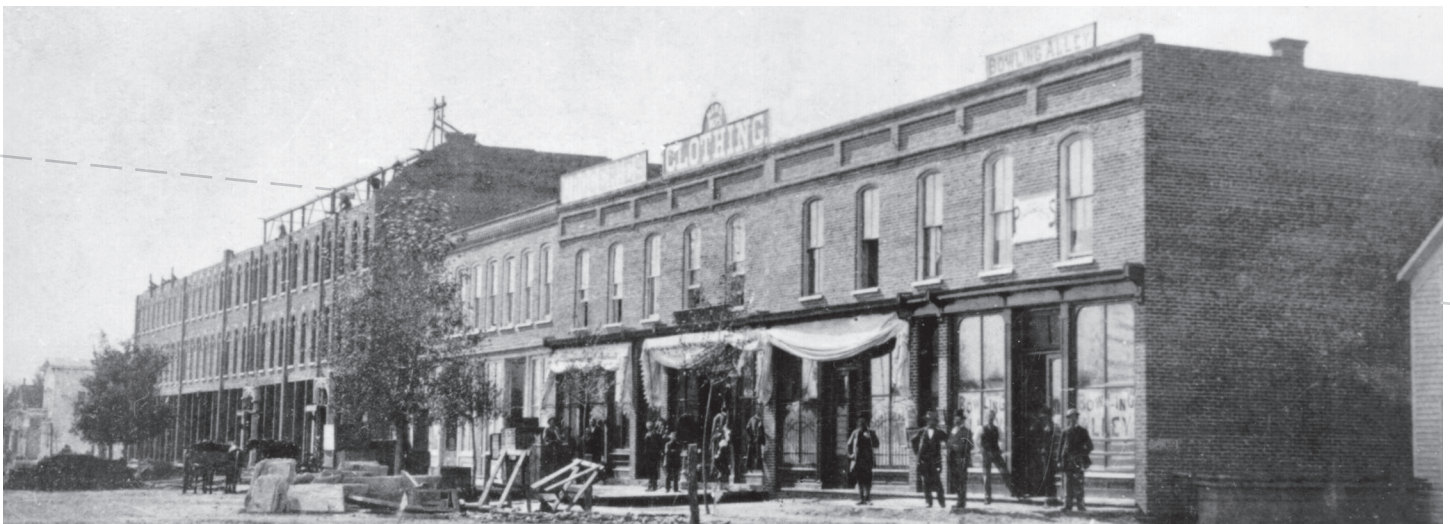
The Opera House under construction on the 100 block of North College Avenue in 1880.
