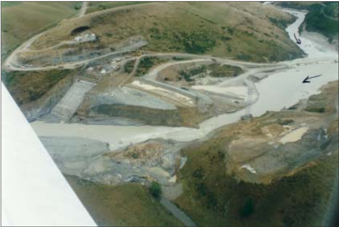
Figure 1. Opuha Dam after the collapse, 6 February 1997.
