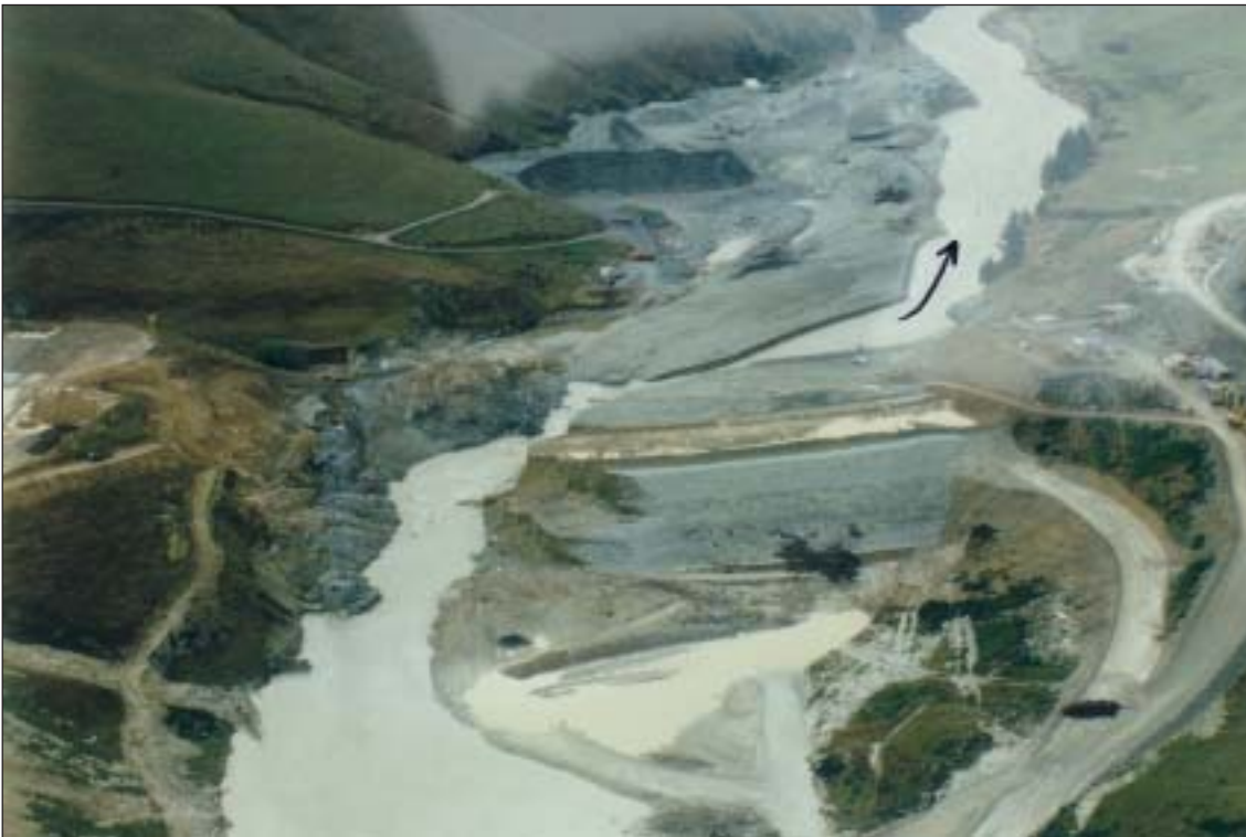
Figure 4. Opuha Dam, looking downstream, 6 February 1997.
