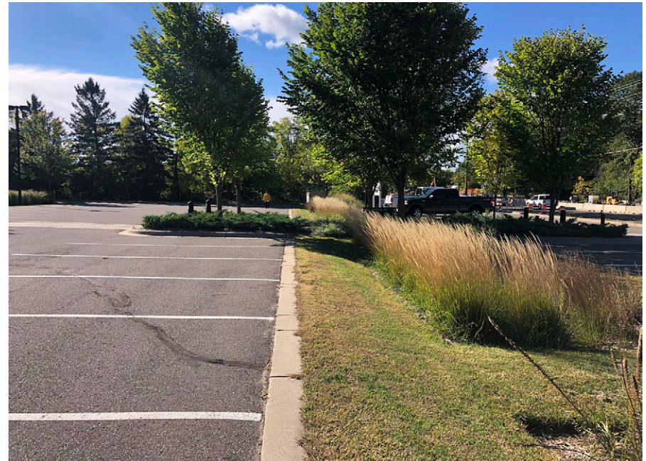
A bioswale includes gentle grades and low-growing vegetation, which fits the parking lot site in Minneapolis, MN.
