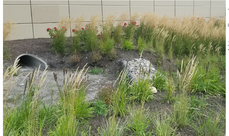
Example of erosion and sediment build up in pretreatment area. Erosion near inlet has exposed geotextile fabric.
