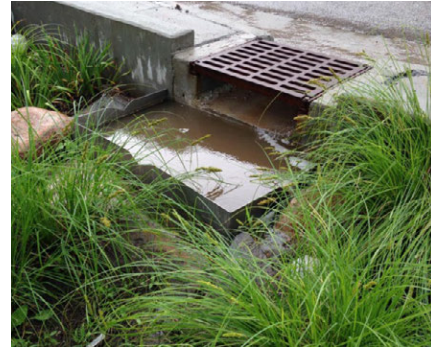
Curb Well Forebay (City of Omaha)
