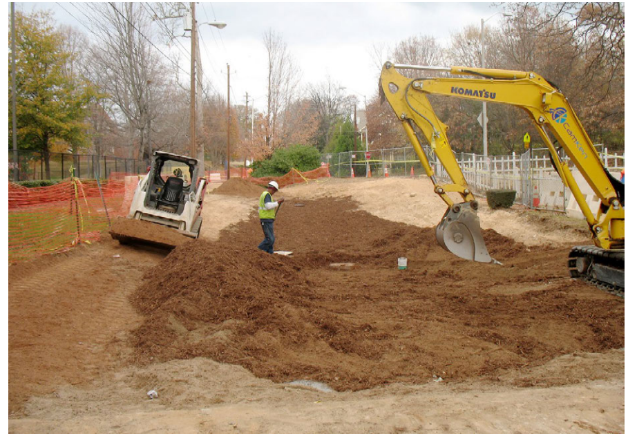
Bioretention facility under construction in Atlanta, GA.
