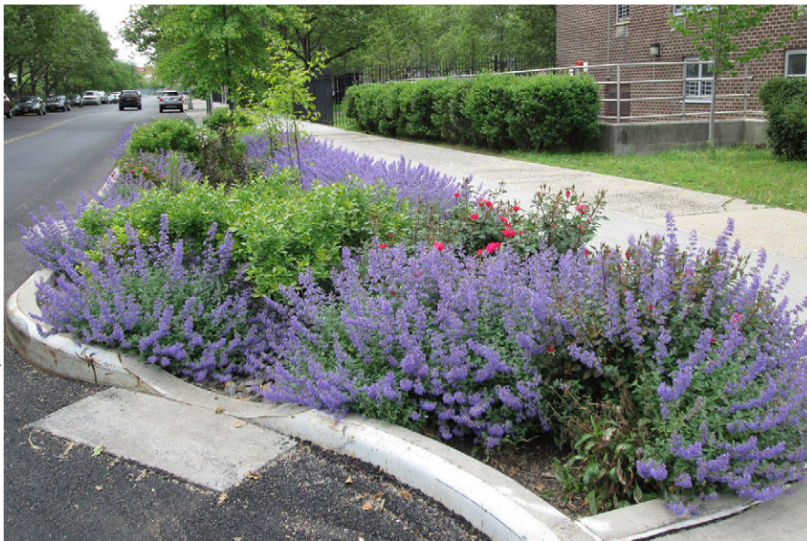
Stormwater curb extension in New York City, NY.
