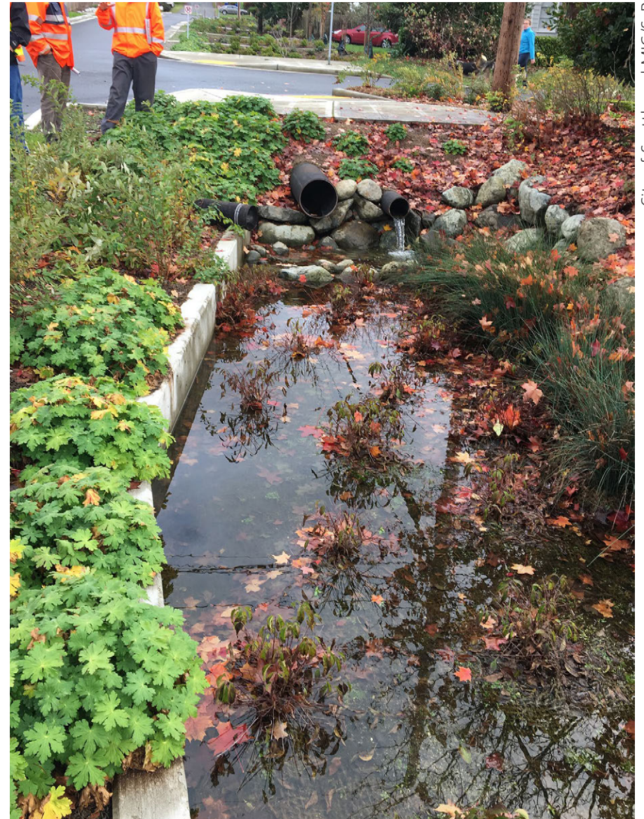
A pipe under a street conveys runoff between bioretention practices in Seattle, WA.
