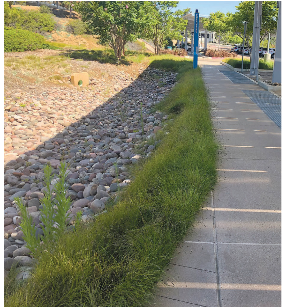
Dense low plantings discourage people from walking into this facility in San Diego, CA.
