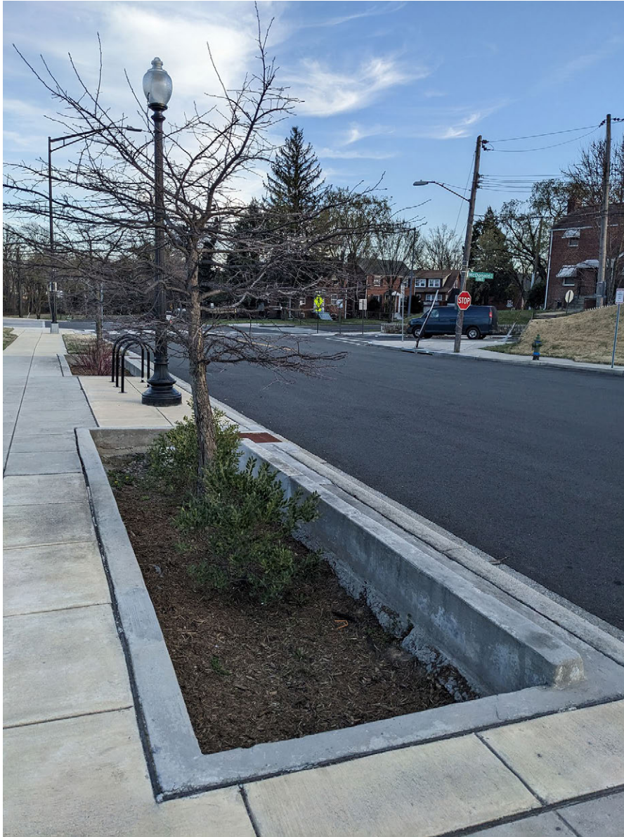
A street-side bioretention planter in Washington, DC.
