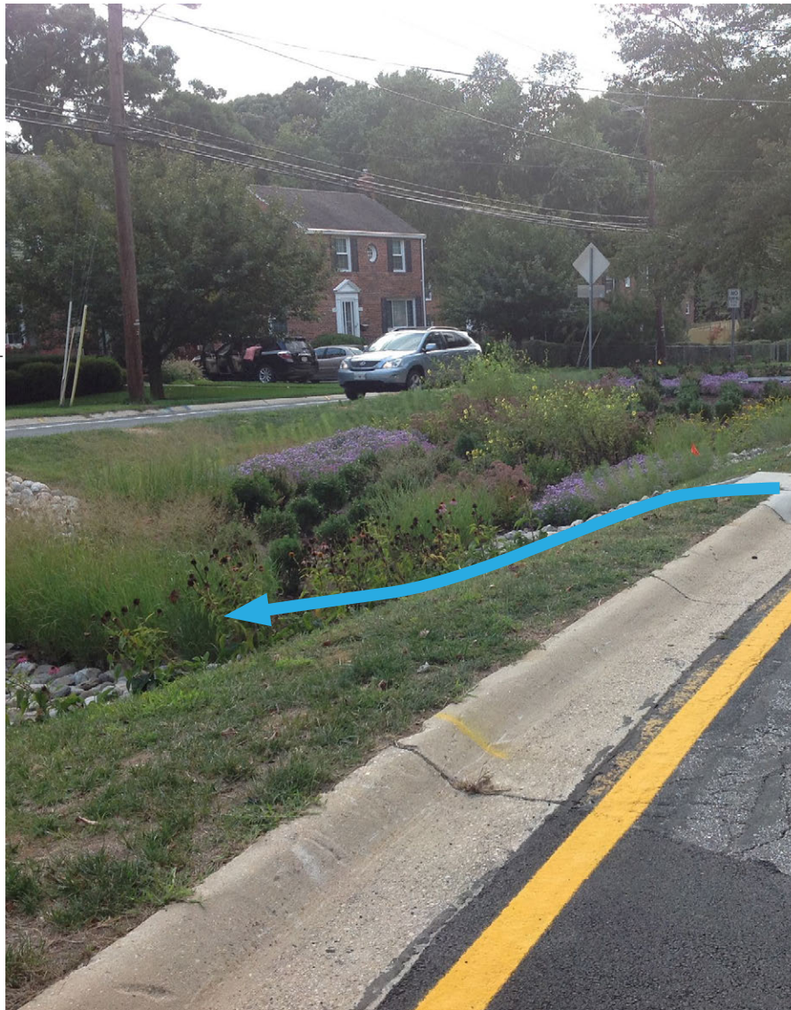
A bioretention practice with side slopes in Montgomery County, MD.
