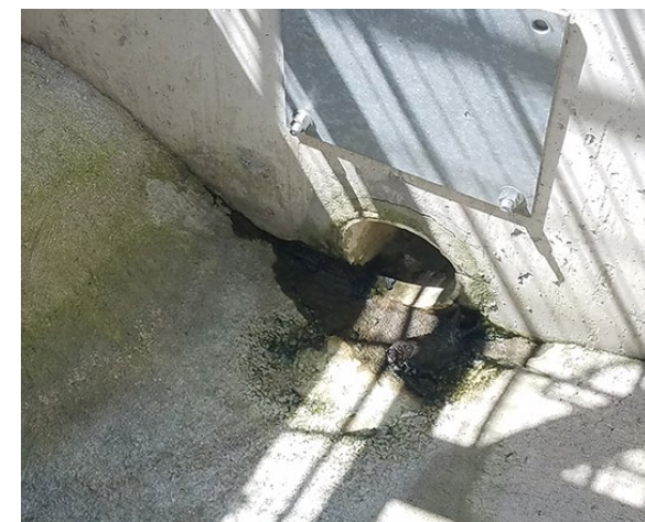
Underdrain outlet in an outlet box.
