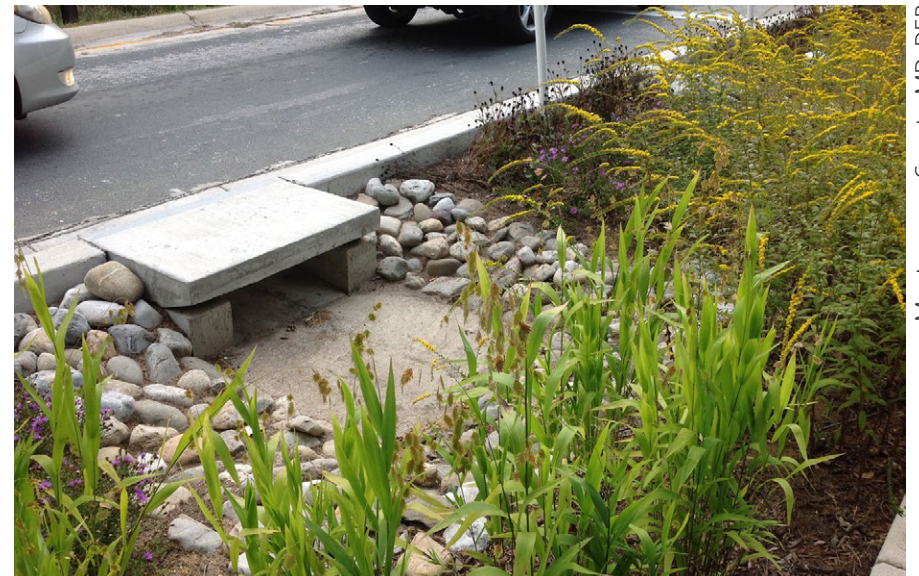
Retrofitted inlet in Montgomery County, MD.
