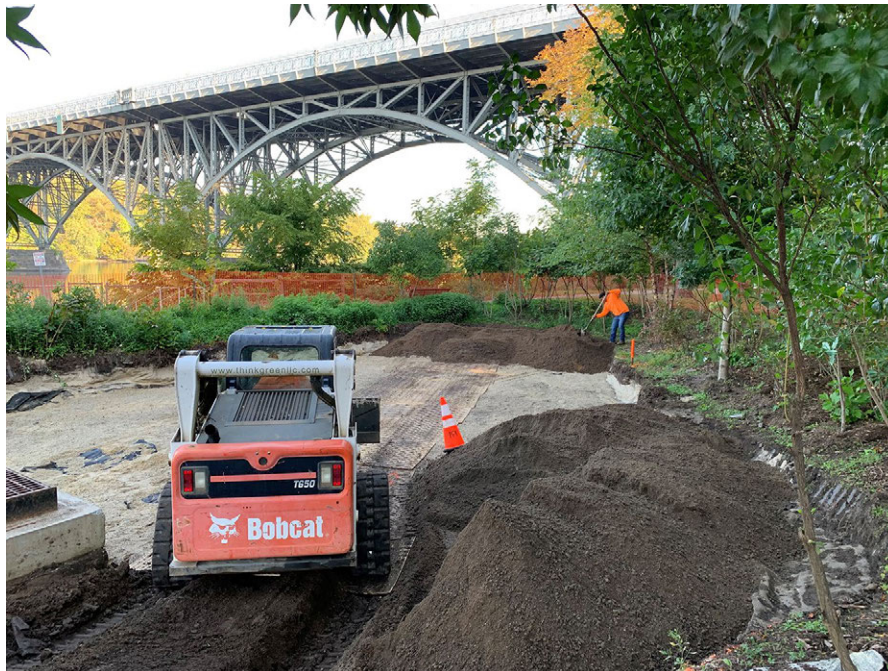
Soilless Soil Initiative project site during construction.
