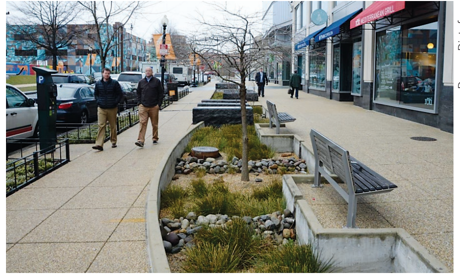
Bioretention with low fencing and walls for safety and benches for pedestrians in Washington, DC.
