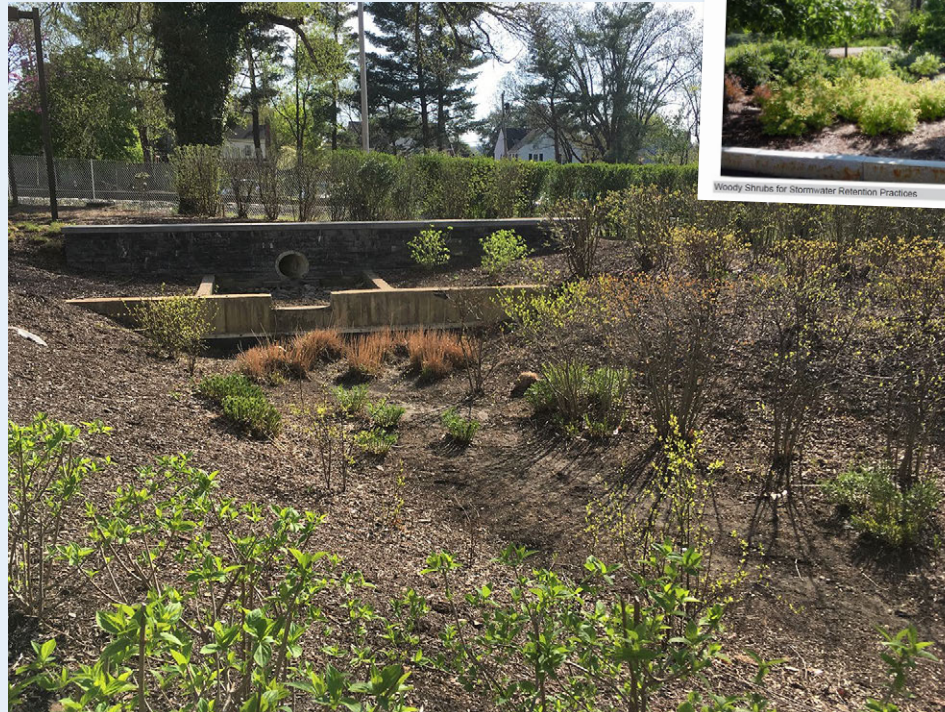
Grasses and woody shrubs in this bioretention facility offer visual interest on the James Madison University campus in Harrisonburg, VA.
