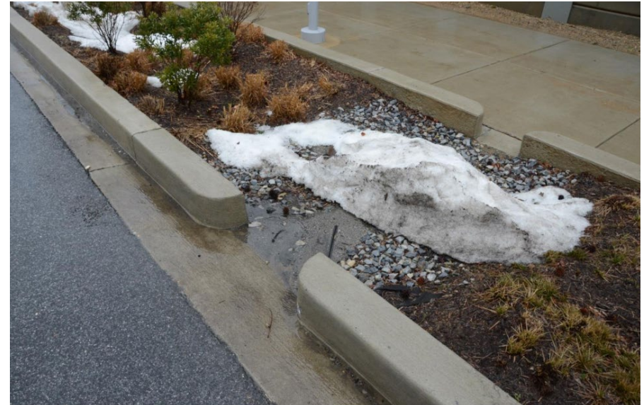
An angled inward curb cut in Washington, DC.
