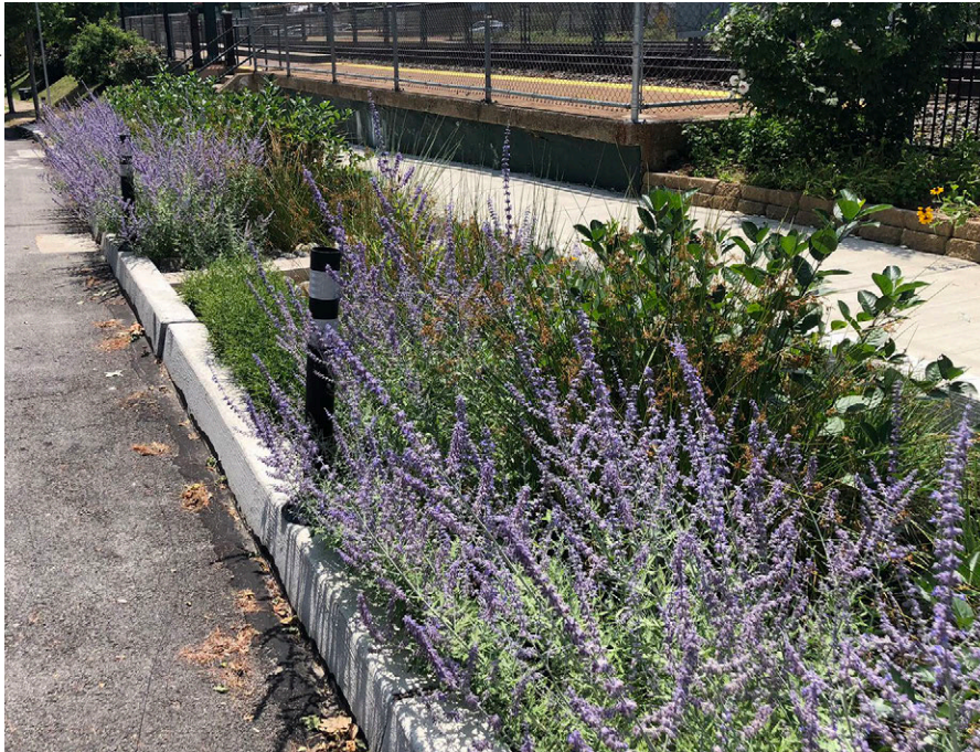
Stormwater curb extension bioretention in Philadelphia, PA.
