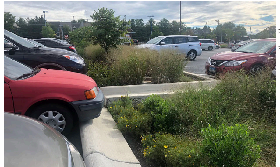
A bioretention practice includes a pedestrian bridge for foot traffic access to a parking lot in Montgomery County, MD.
