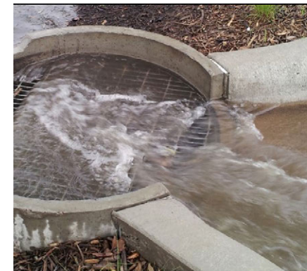
Inlet Sump (ACF Environmental)
