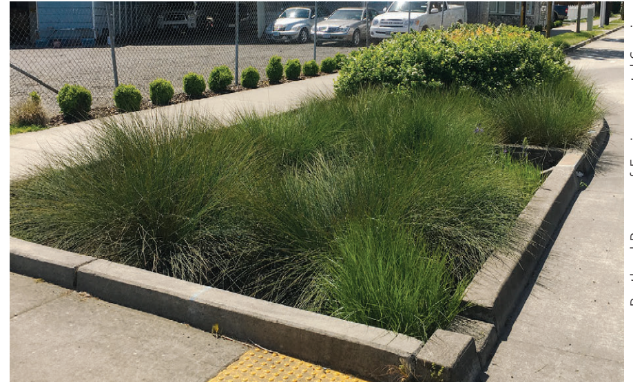
Aesthetically pleasing naturalized vegetation in a pedestrian area in Portland, OR.
