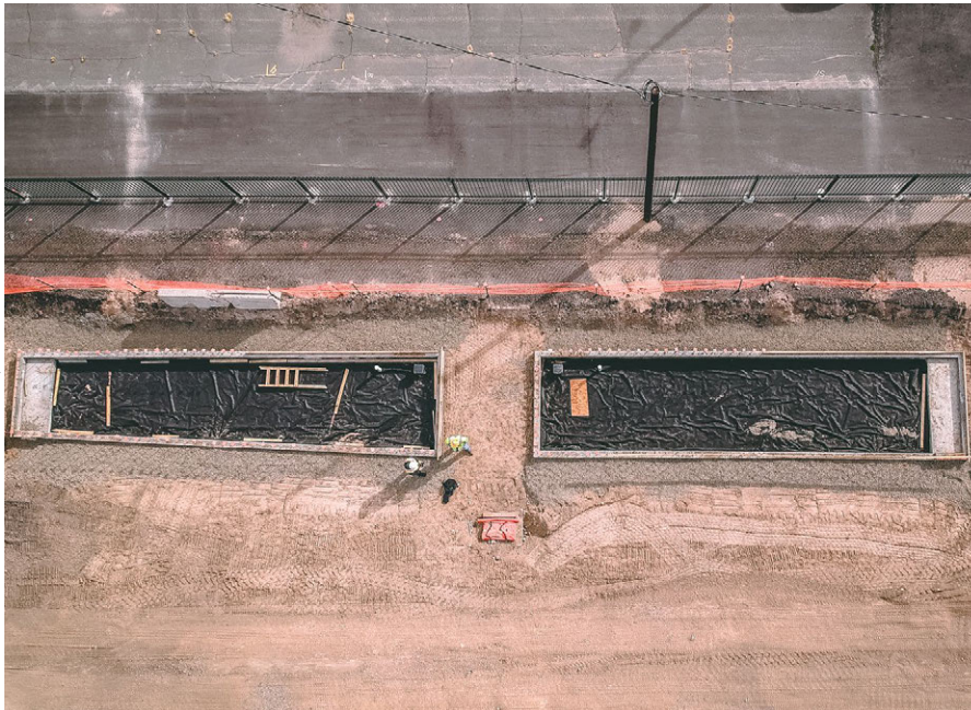
Aerial image showing impermeable liners at the bottom of two bioretention cells under construction in Denver, CO.
