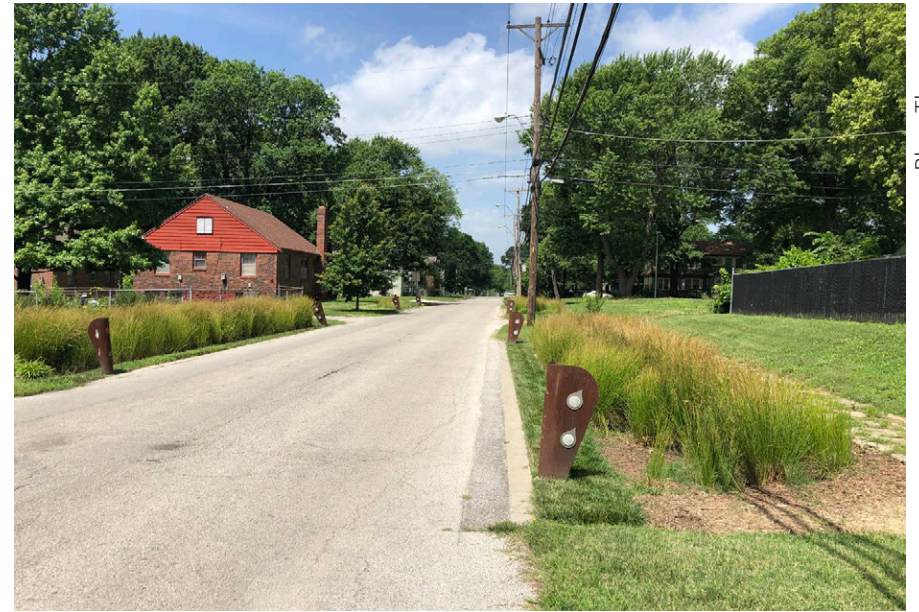
Curbless bioretention in Kansas City, MO.
