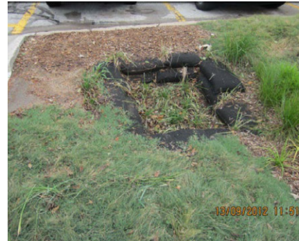
Vegetated Bag Forebay (City of Omaha)
