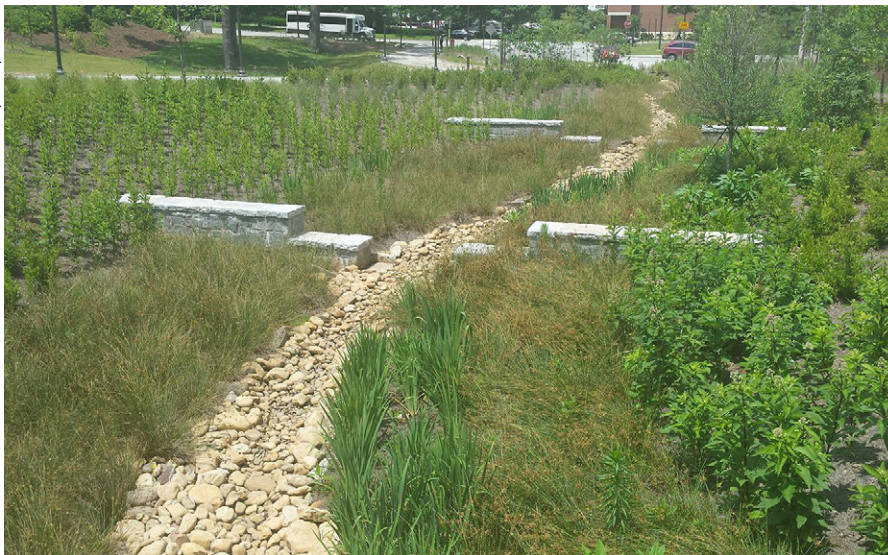
Similar species are grouped in this bioretention practice in Atlanta, GA.
