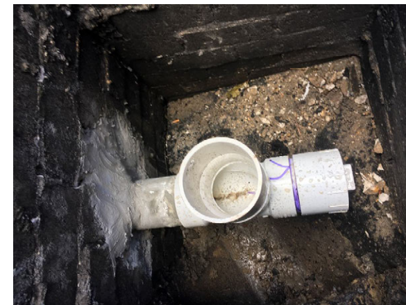
An IWS system with an outlet box.
