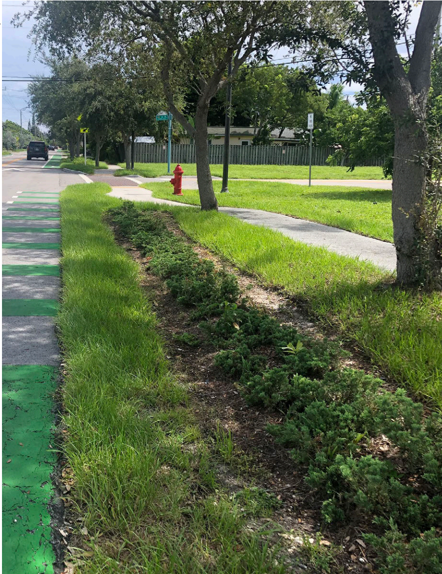
Curbside bioretention with a VFS that treats sheet flow in Fort Lauderdale, FL.
