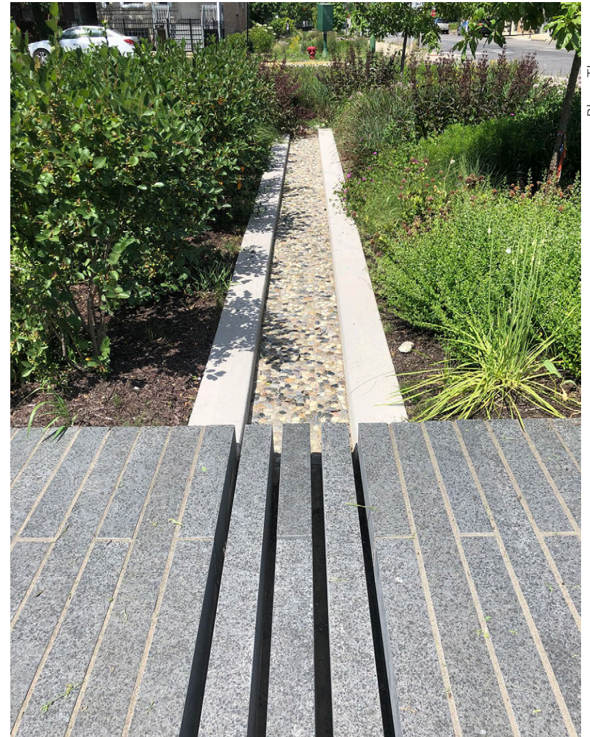
The City of Chicago installed a decorative trench drain with a walkway to allow users to see water flowing through this facility. In an area traditionally lacking investment, this allows community members to connect with nature and beautifies the surrounding areas as well.
