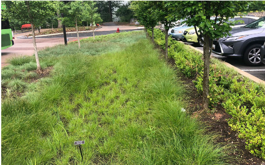
Bioretention with low-height plants in a parking lot in Montgomery County, MD.
