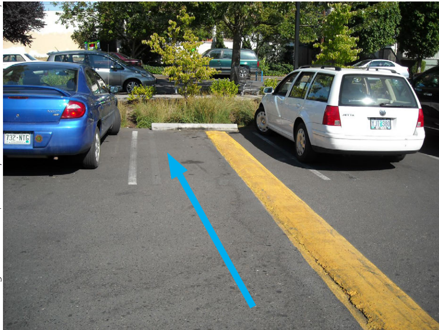
A speed bump intercepts and redirects runoff.
