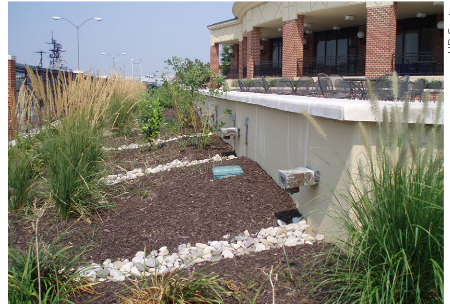
An infiltration planter treats runoff while adding aesthetic value to an outdoor space at the Navy Yard in Washington, DC.
