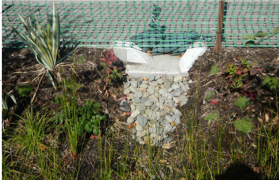
A depressed curb cut in Seattle, WA.
