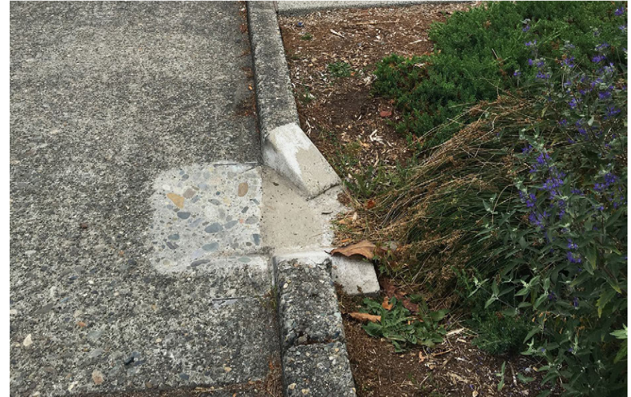
An angled curb cut in Seattle, WA.
