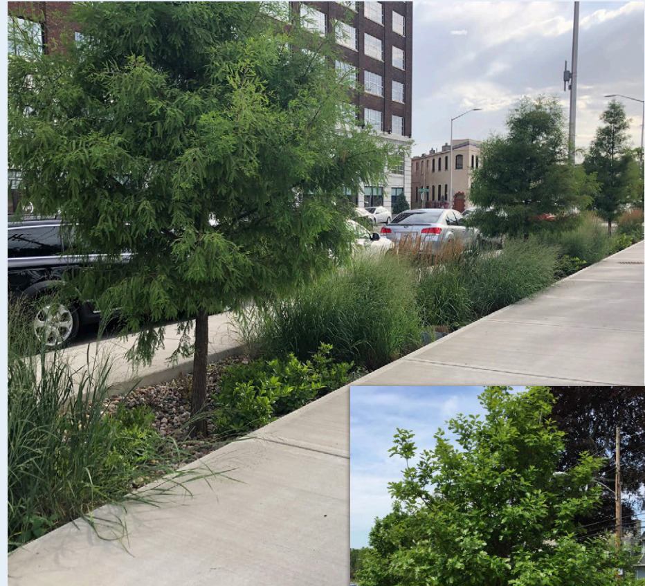
Bioretention facility with trees in Kansas City, MO.
