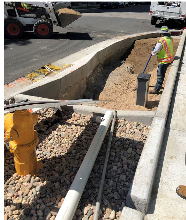
Installing BSM amended with biochar, zeolite, and coconut coir in Denver, CO.
