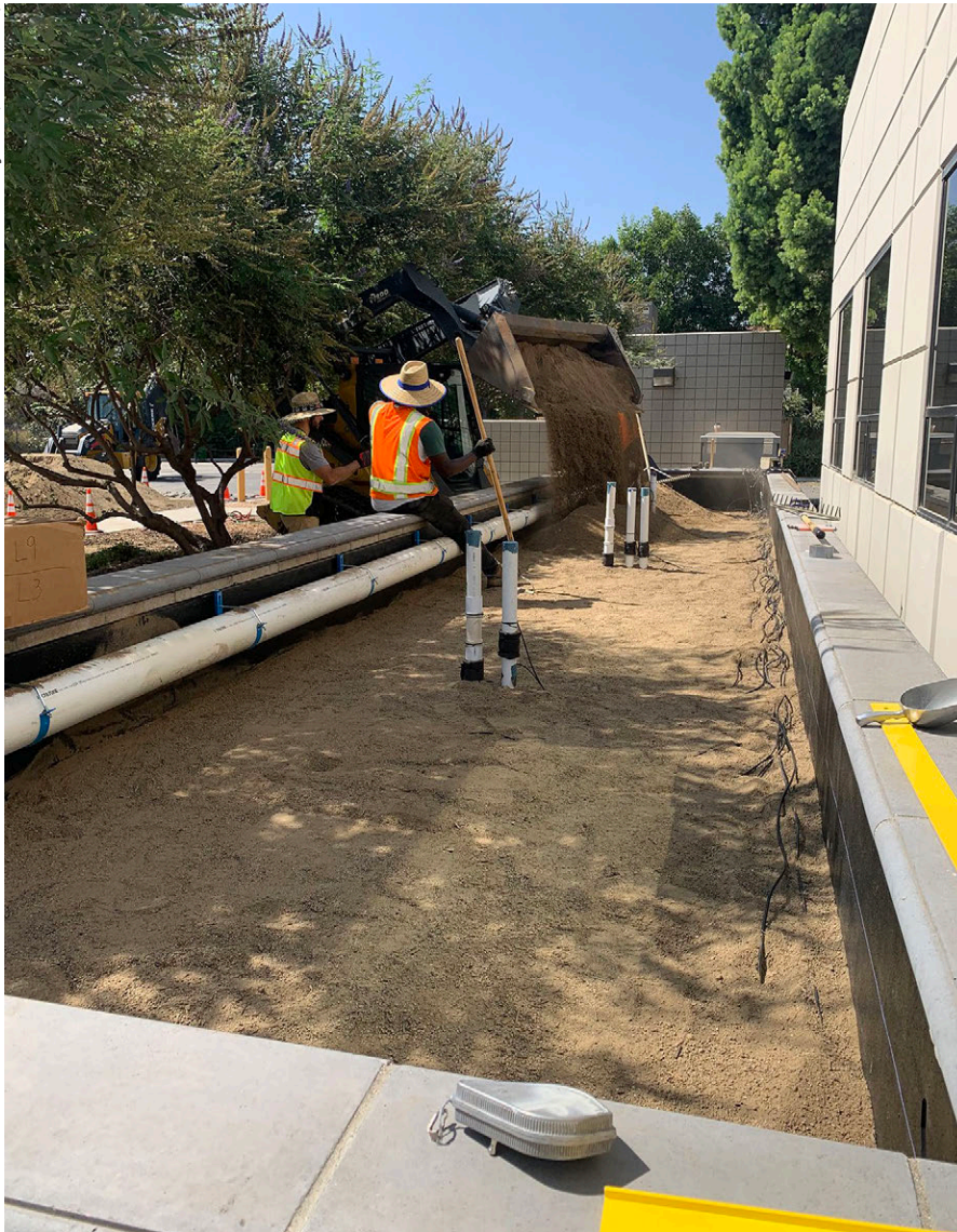
BSM installation for a bioretention planter implemented by the Riverside County Flood Control and Water Conservation District, Riverside, CA.
