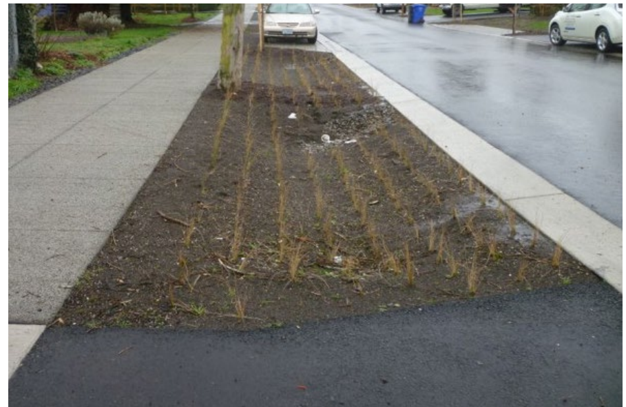
Curbside bioretention with a level spreader in Portland, OR.
