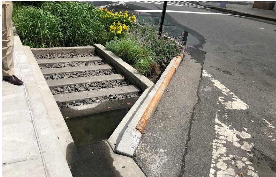
Concrete forebay in New York City, NY.
