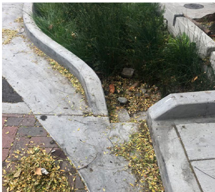
Curb Extension Inlet (Rhea Thompson)
