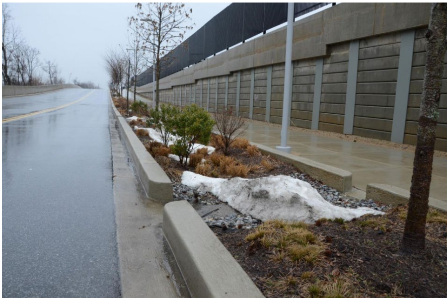
Bioretention can be configured as a series of individual facilities (top) or a single, street-length facility with multiple inlets (bottom).
