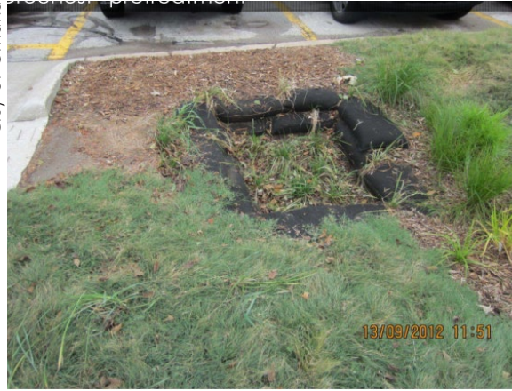
A vegetated bag forebay in Omaha, NE.
