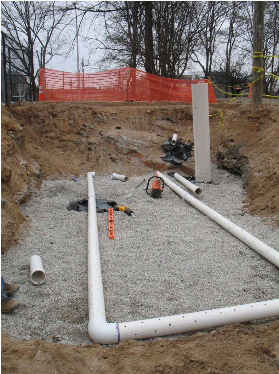
Underdrains being installed in Atlanta, GA.
