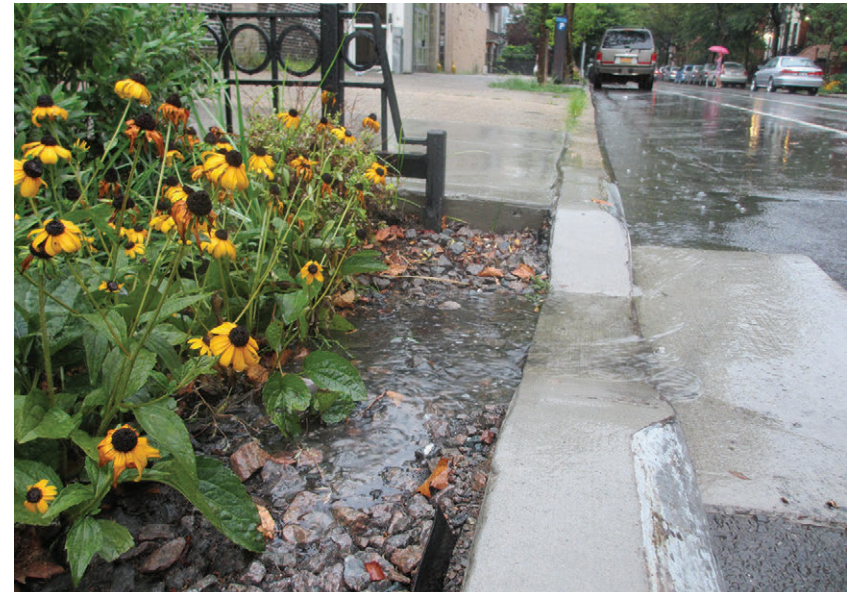
A well-designed inlet.
