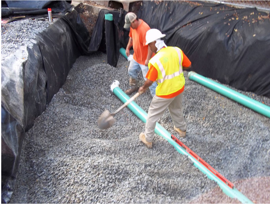
Installing aggregate media in Atlanta, GA.
