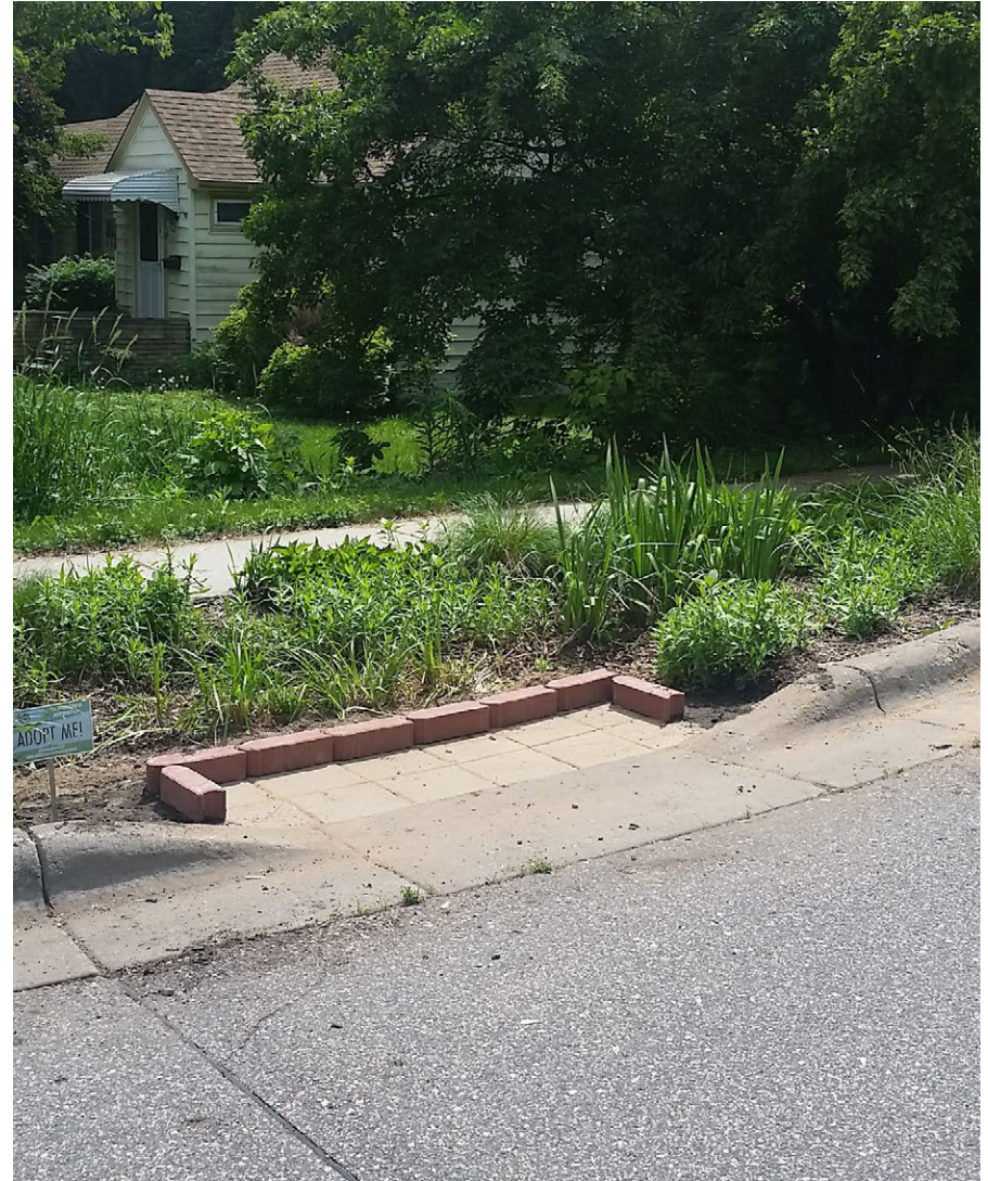
The Middle St. Croix Watershed Management Organization developed this low-cost shallow sump to capture runoff and debris.
