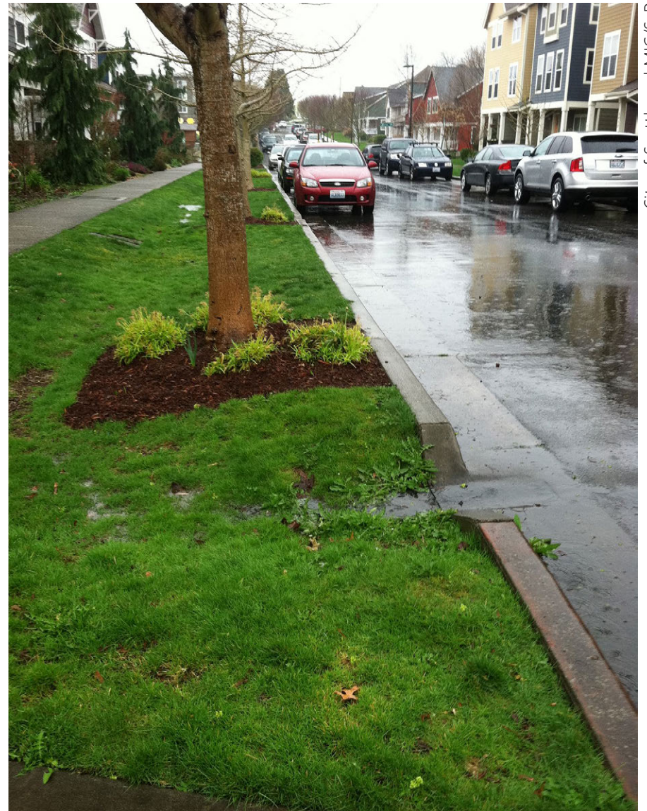
Water flows through a curb cut in Seattle, WA.
