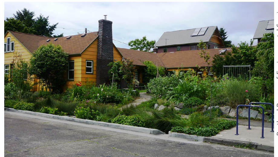
Street-side bioretention in Portland, OR.
