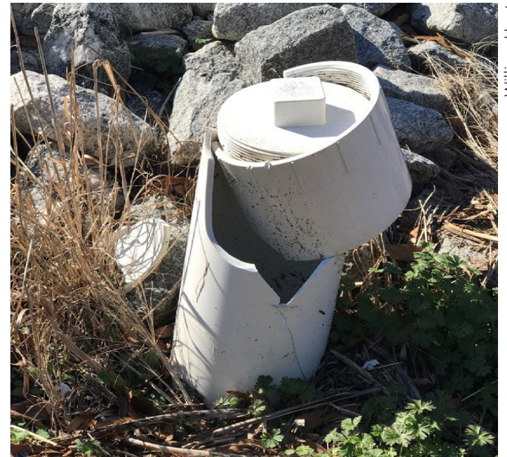
A broken cleanout.
