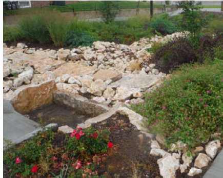
Limestone Forebay (City of Omaha)
