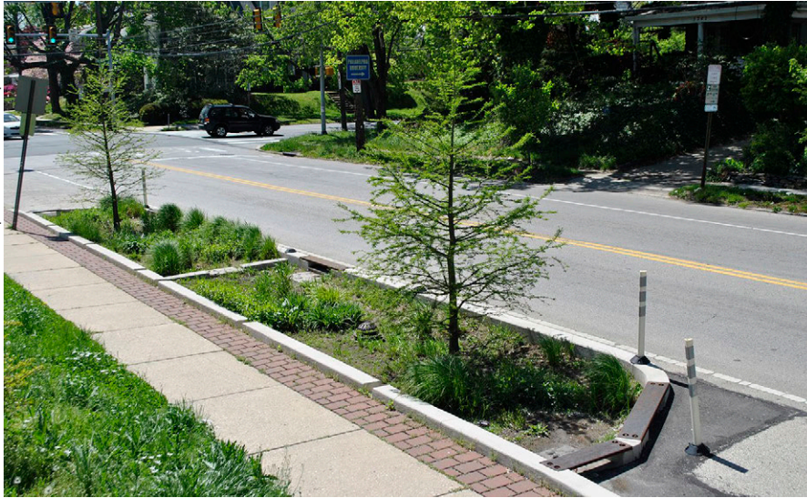
Stormwater curb extension in Philadelphia, PA.
