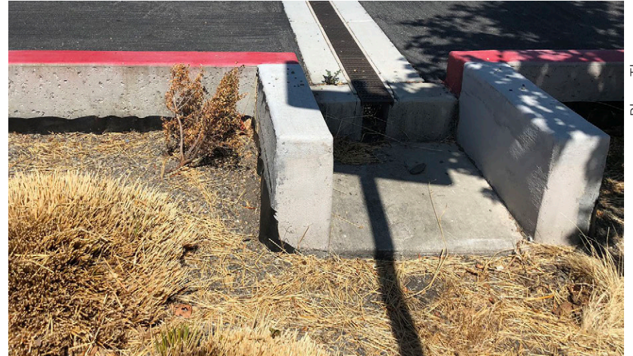
Concrete splash pad in San Mateo, CA
