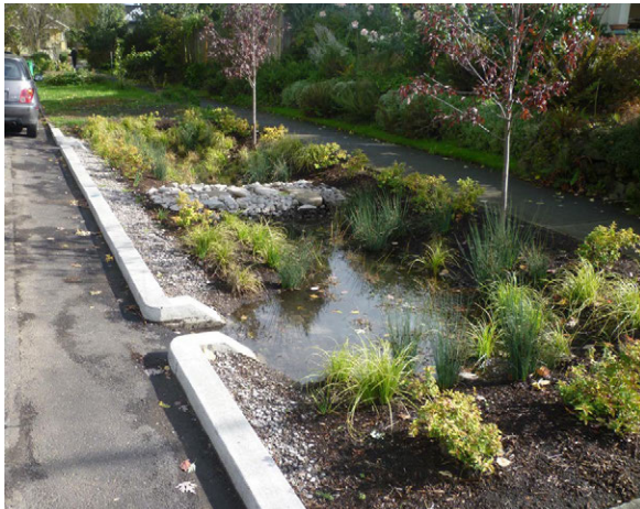
These three bioretention facilities lack proper step-out zones, creating a safety hazard for individuals entering and exiting vehicles. Providing easy access to step-out zones and pathways allow for pedestrian circulation and minimize trampling-related system damage.
