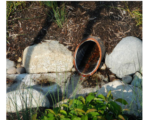
Pipe (City of Seattle and MIG/SvR)
