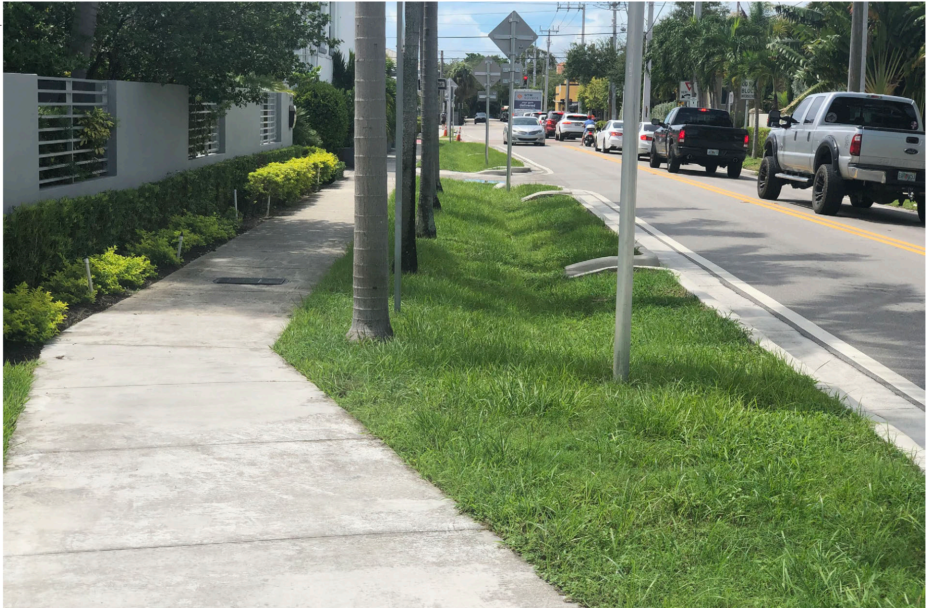
This grassy street-side bioswale is easy to clean and maintain and fits in with the community aesthetic in Fort Lauderdale, FL.
