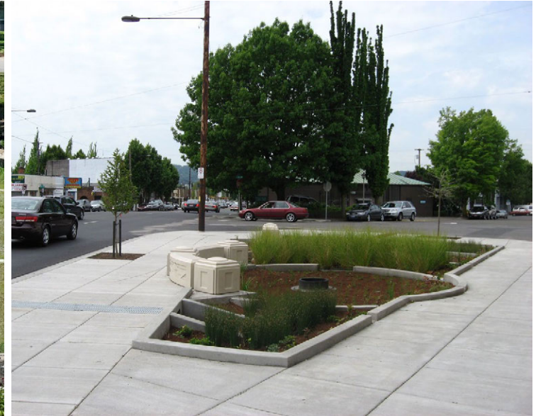
Raised curbs and seating help delineate the edges of the GSI while providing a place for respite in Portland, OR.
