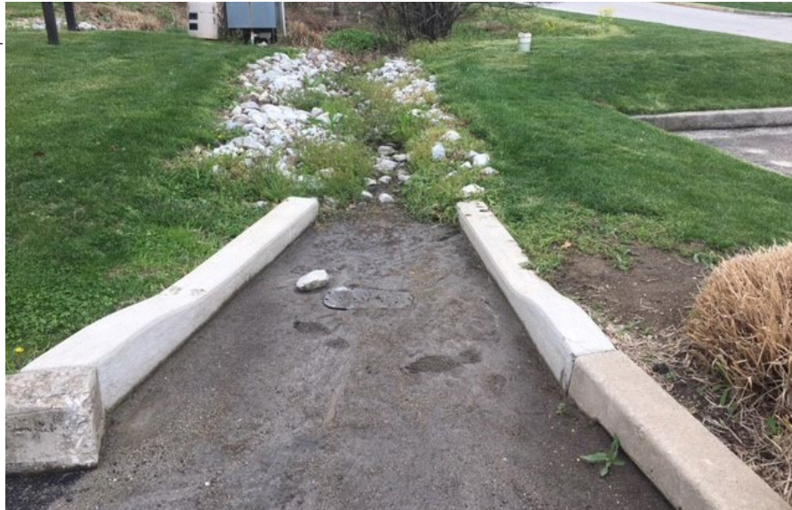
An angled inward curb cut at Villanova University, PA.
