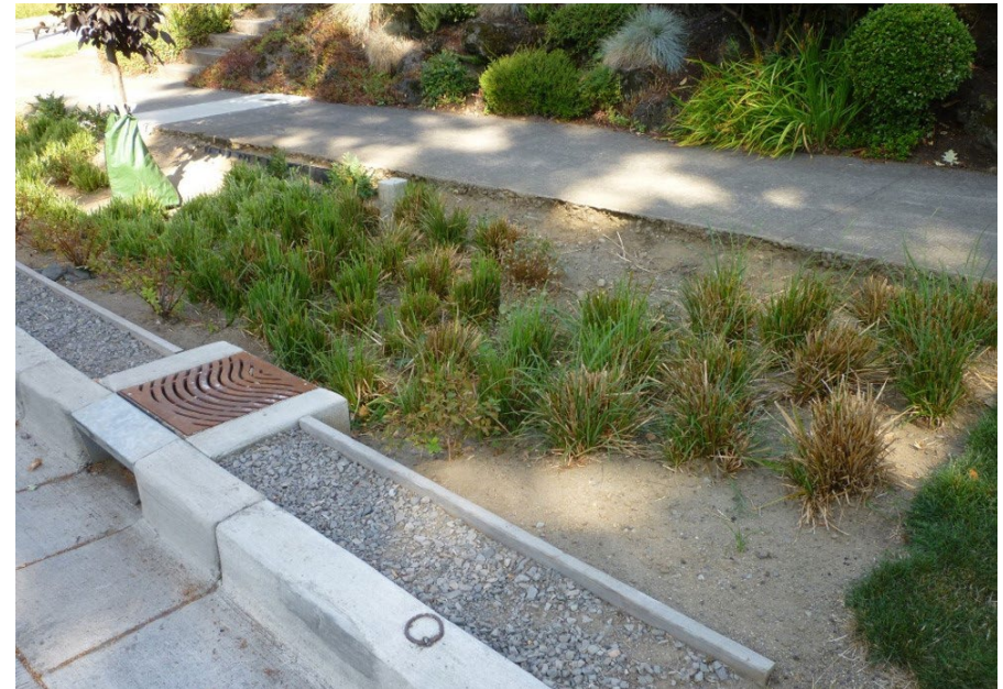
Examples of two step-out zone designs (left, right) in Portland, OR. Concrete is generally preferable over gravel due to weed growth.
