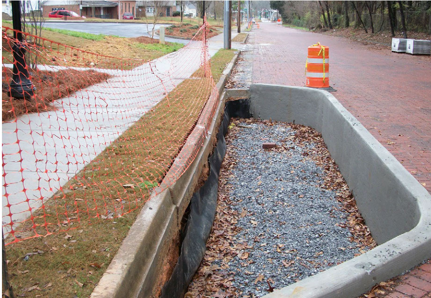
Bioretention under construction in Atlanta, GA.
