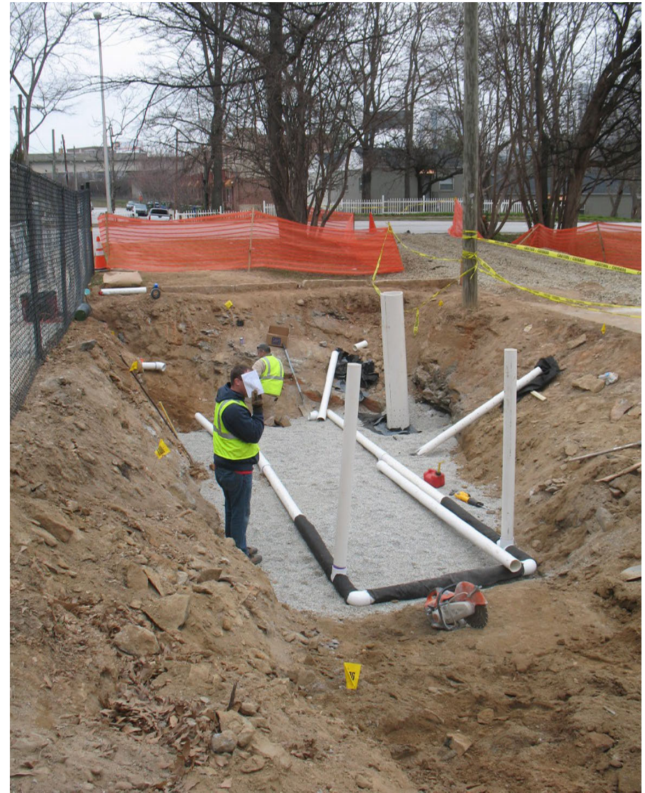
Bioretention under construction in Atlanta, GA.
