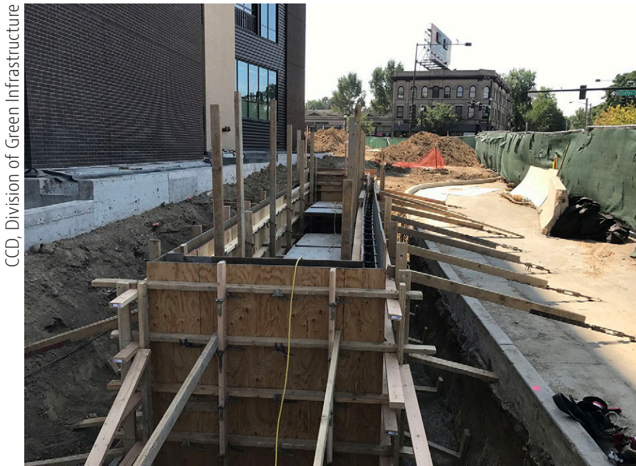
Bioretention under construction in Denver, CO.
