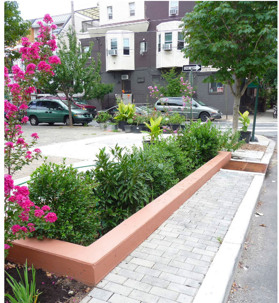
A raised curb edge delineates a facility in Philadelphia, PA.
