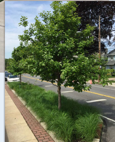
Bioretention facility with trees in Philadelphia, PA.
