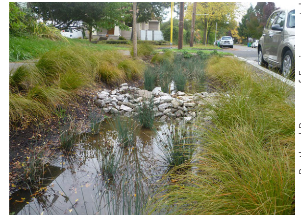
Rock check dam in a bioretention facility in Portland, OR.
