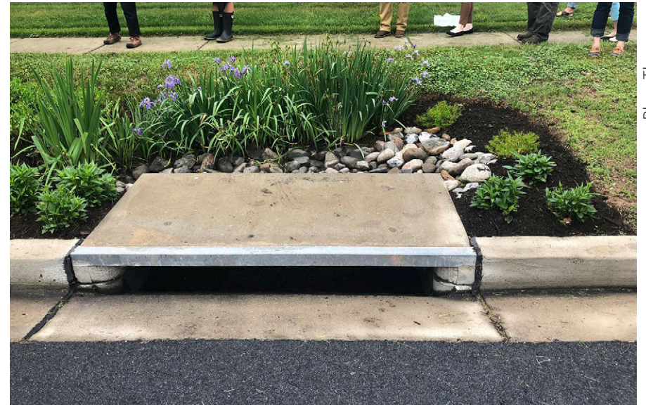
Retrofitted inlet in Montgomery County, MD.
