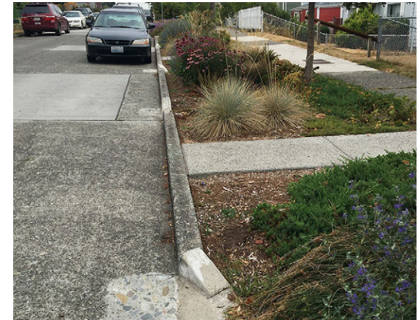
These three bioretention facilities lack proper step-out zones, creating a safety hazard for individuals entering and exiting vehicles. Providing easy access to step-out zones and pathways allow for pedestrian circulation and minimize trampling-related system damage.
