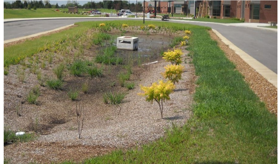
Curbside bioretention with a level spreader and VFS in Omaha, NE.
