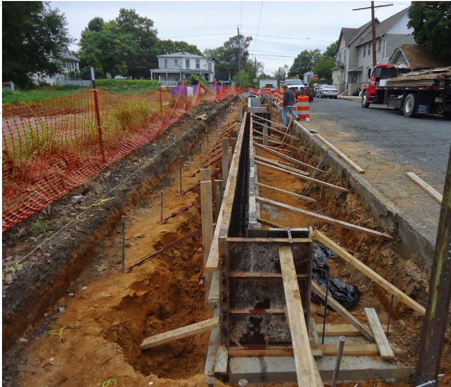
Bioretention under construction in Camden, NJ.
