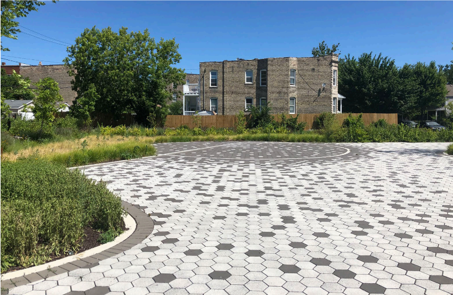
Permeable pavers were installed around this bioretention facility to create a stage and event space for the community in Chicago, IL.
