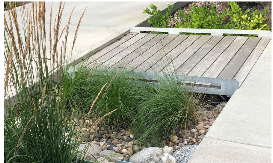
A bioretention practice designed with a pedestrian bridge in Kansas City, MO.
