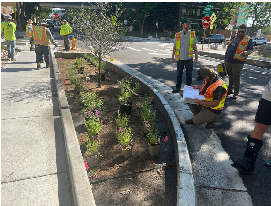
Staff follow a plan as they prepare potted bushes and grasses for planting. Potted plants offer instantaneous aesthetic appeal and can better tolerate irregular watering during establishment.
