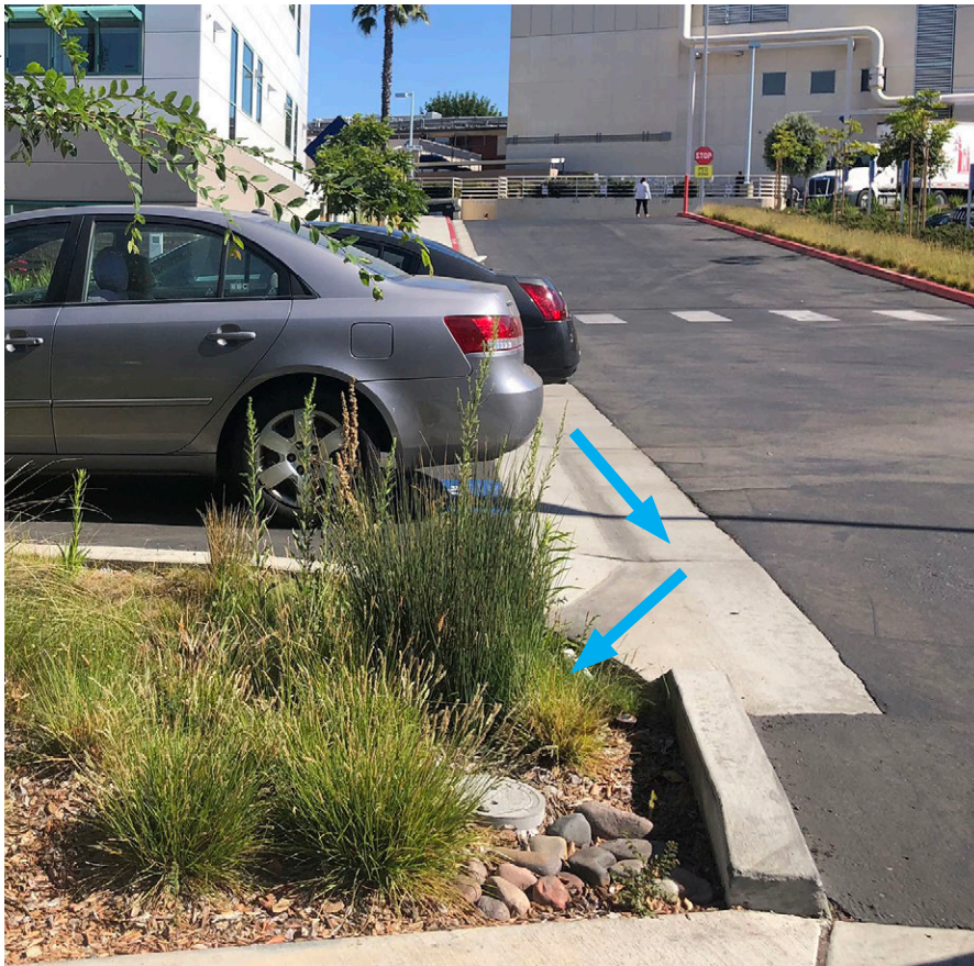
A runnel directs runoff to a bioretention practice in San Diego, CA.
