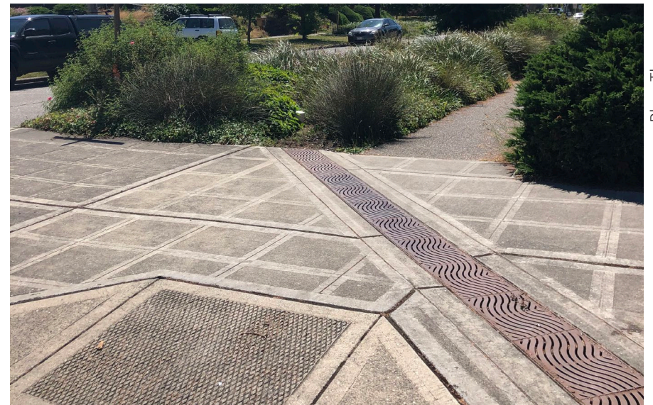
A trench drain allows for runoff conveyance and pedestrian circulation in Seattle, WA.
