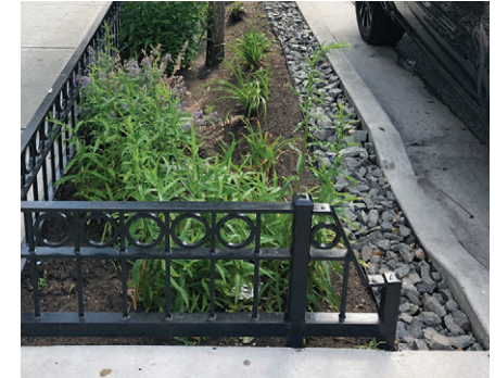
Gravel Forebay (Rhea Thompson)
