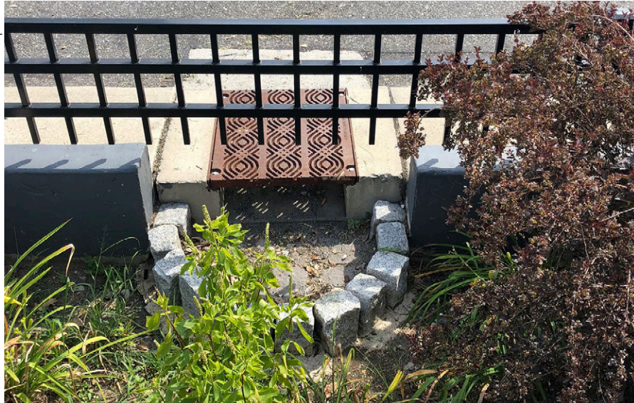
Concrete forebay in New York City, NY.
