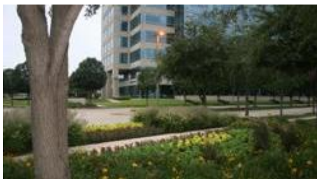
The Granite Park office complex reduced its irrigation water use by about 40 percent after installing a WaterSense labeled weather-based controller and other upgrades.
