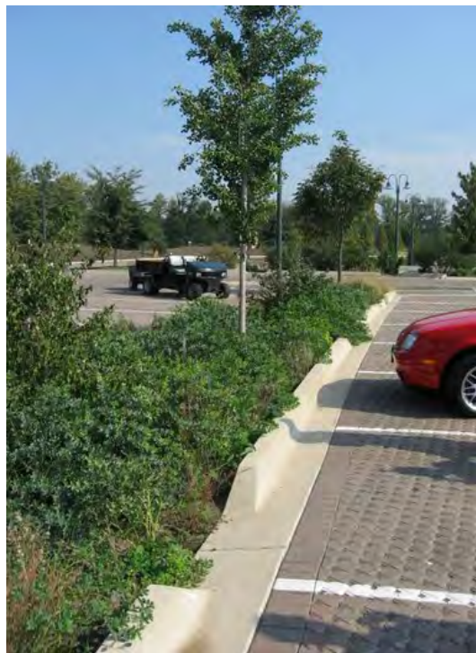
Figure 4. Parking lot bioswale and permeable pavers in Chicago.
