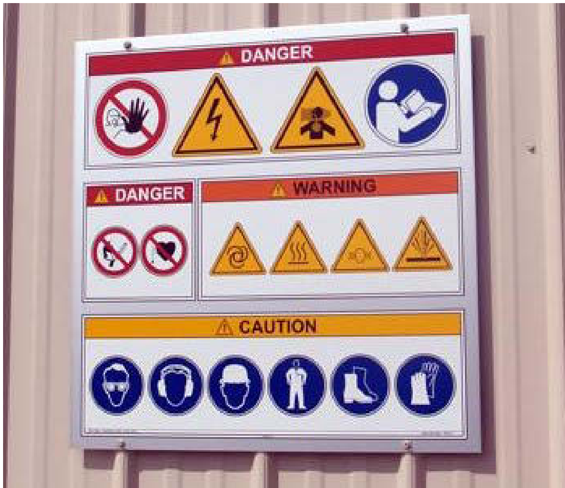
Figure 11.2. Safety Signage on AD System 62
