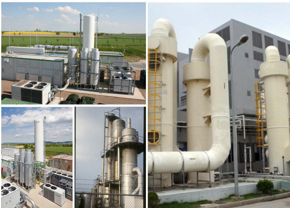
Figure 5.4. Process Equipment Used to Remove Biogas Impurities When Upgrading 45
