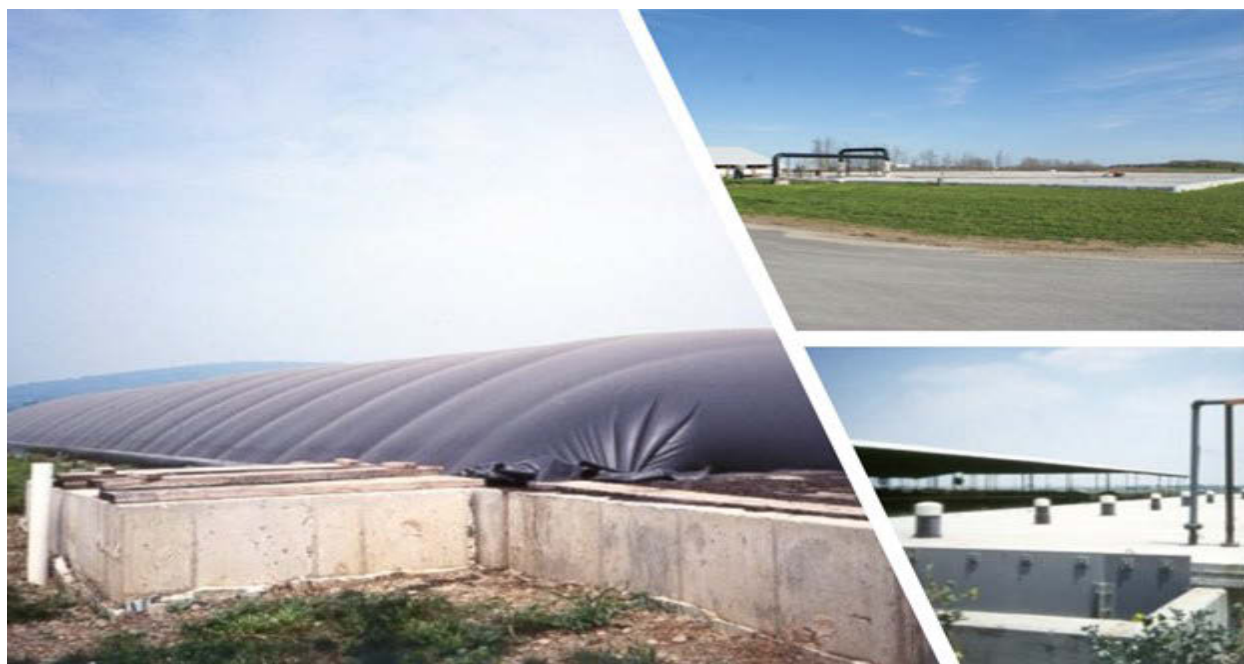
Figure 3.9. Examples of Plug-flow Digesters 27
