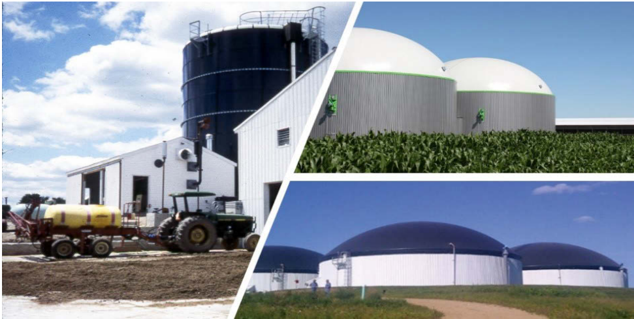
Figure 3.11. Examples of Complete Mix Digesters 29
