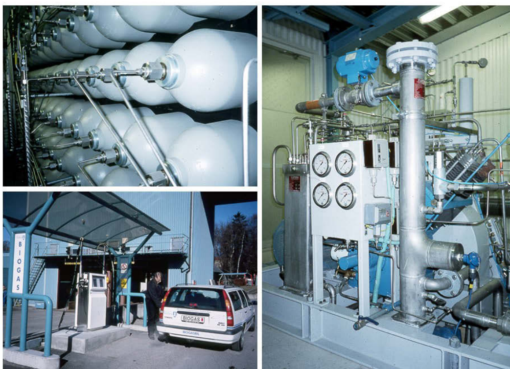
Figure 5.5. Centralized Digester Producing R-CNG for City Fleet
