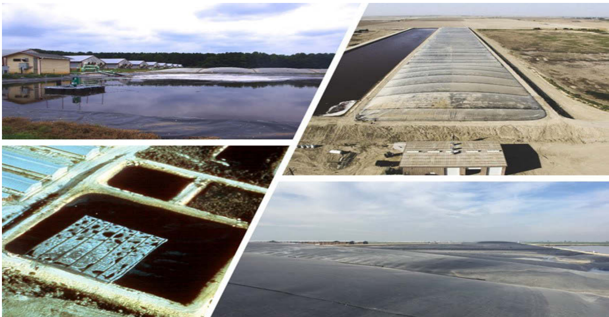
Figure 3.7. Examples of Covered Anaerobic Lagoons 25
