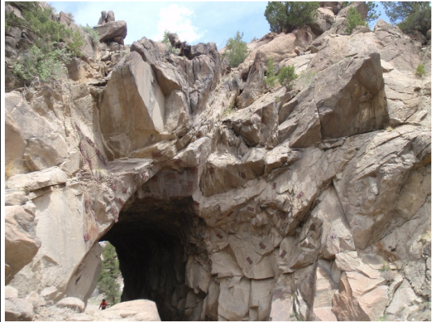
Condition State 3 Unfavorable joint orientation with open joints
