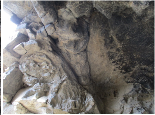
Condition State 3 Converging open joints
