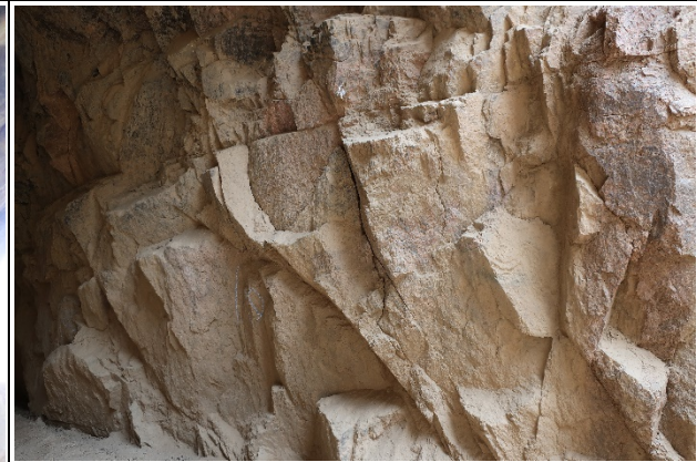
Condition State 3 Converging open joints
