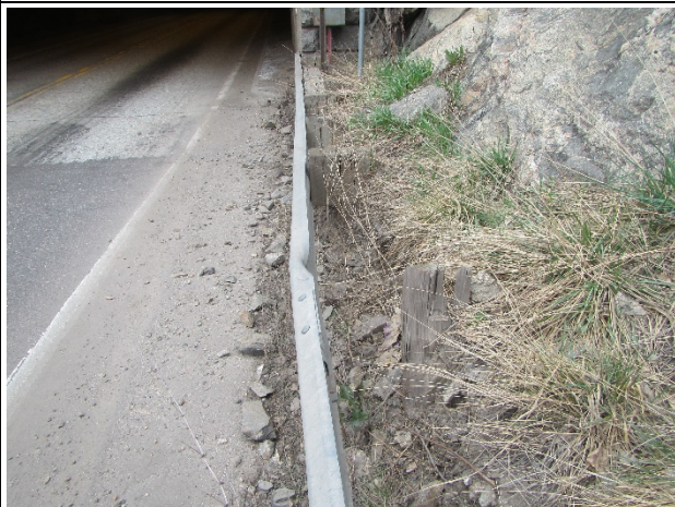
Condition State 4 Broken posts and damaged rail
