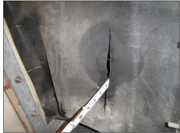
Condition State 2 Tear in fan diaphragm
