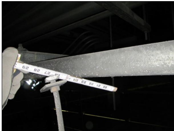
Condition State 4 Disconnected hanger rod
