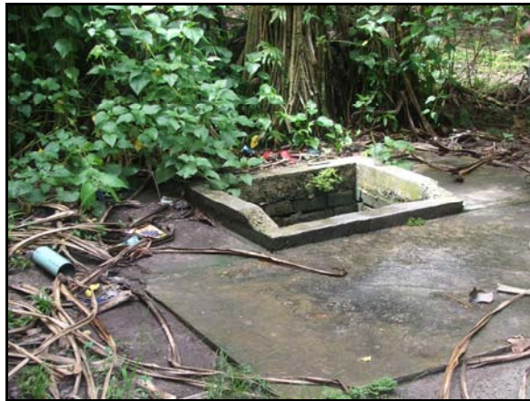
Figure 3. Hand-dug wells on Ulithi (A and B) and Pingelap (C and D). The depth to water in the wells ranges from 2 to 3 m, and also fluctuates with the rise and fall of the tides. The water within the wells is used mainly for bathing and washing clothes, and is extracted by either a rope and bucket or a small electric pump. Normally a well is shared by several households. Most wells are lined with concrete or rocks.
