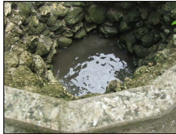
Figure 3. Hand-dug wells on Ulithi (A and B) and Pingelap (C and D). The depth to water in the wells ranges from 2 to 3 m, and also fluctuates with the rise and fall of the tides. The water within the wells is used mainly for bathing and washing clothes, and is extracted by either a rope and bucket or a small electric pump. Normally a well is shared by several households. Most wells are lined with concrete or rocks.
