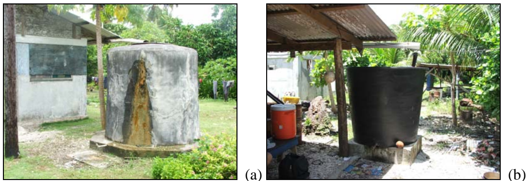
Figure 2. Roof catchments on Falalop Island, Ulithi Atoll, Yap State, FSM. Most households have their own catchment tank. The water from the tanks is used for drinking, cooking, and washing dishes. The tanks vary in construction material and size. Older tanks (a) are made from concrete, while newer ones (b) are made from fiber glass.
