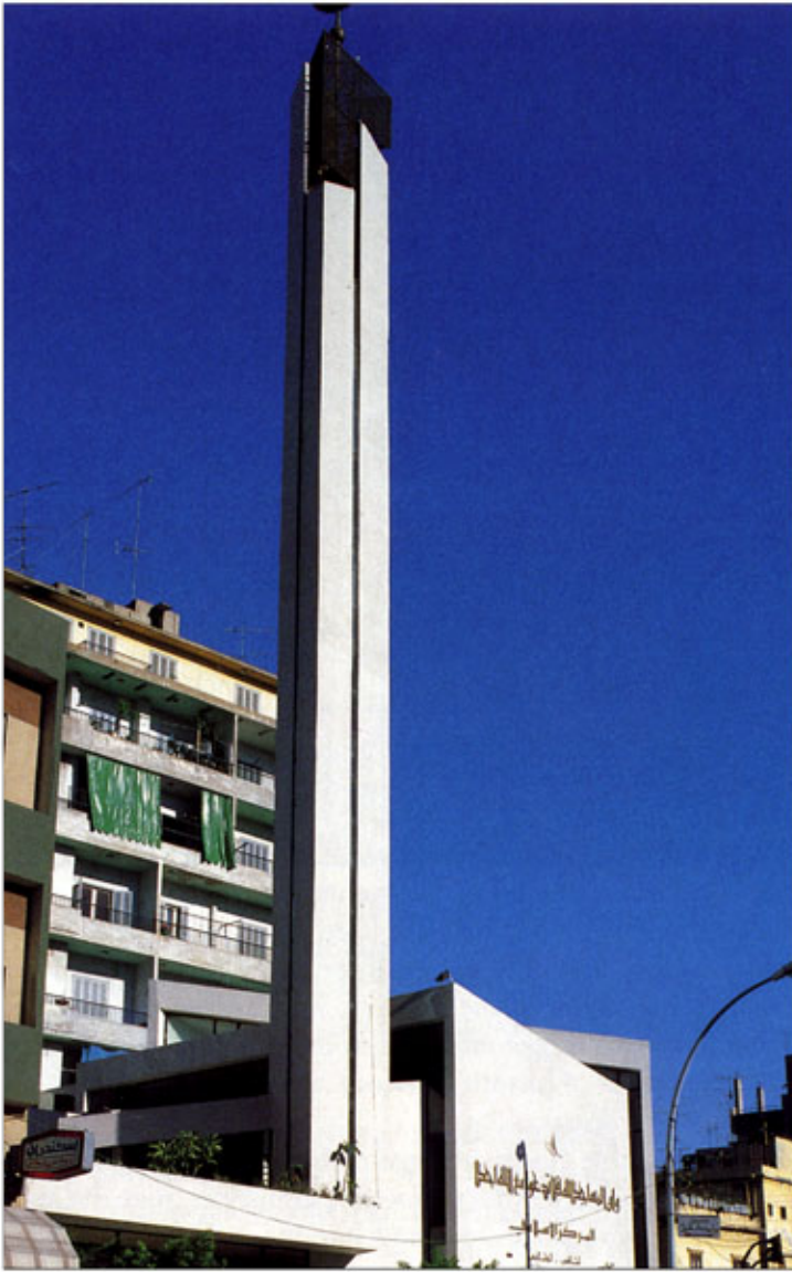
Plan of State Mosque, Kuwait City, Kuwait (left). The design is for a new classic Islamic type of mosque. Aysha Bakkar Mosque, Beirut, Lebanon (above), and a mosque in Abu Dhabi (right). The first is representative of the contemporary/modern trend, while the second is a clear-cut example of the eclectic/Arabian Nights tendency in mosque design.
