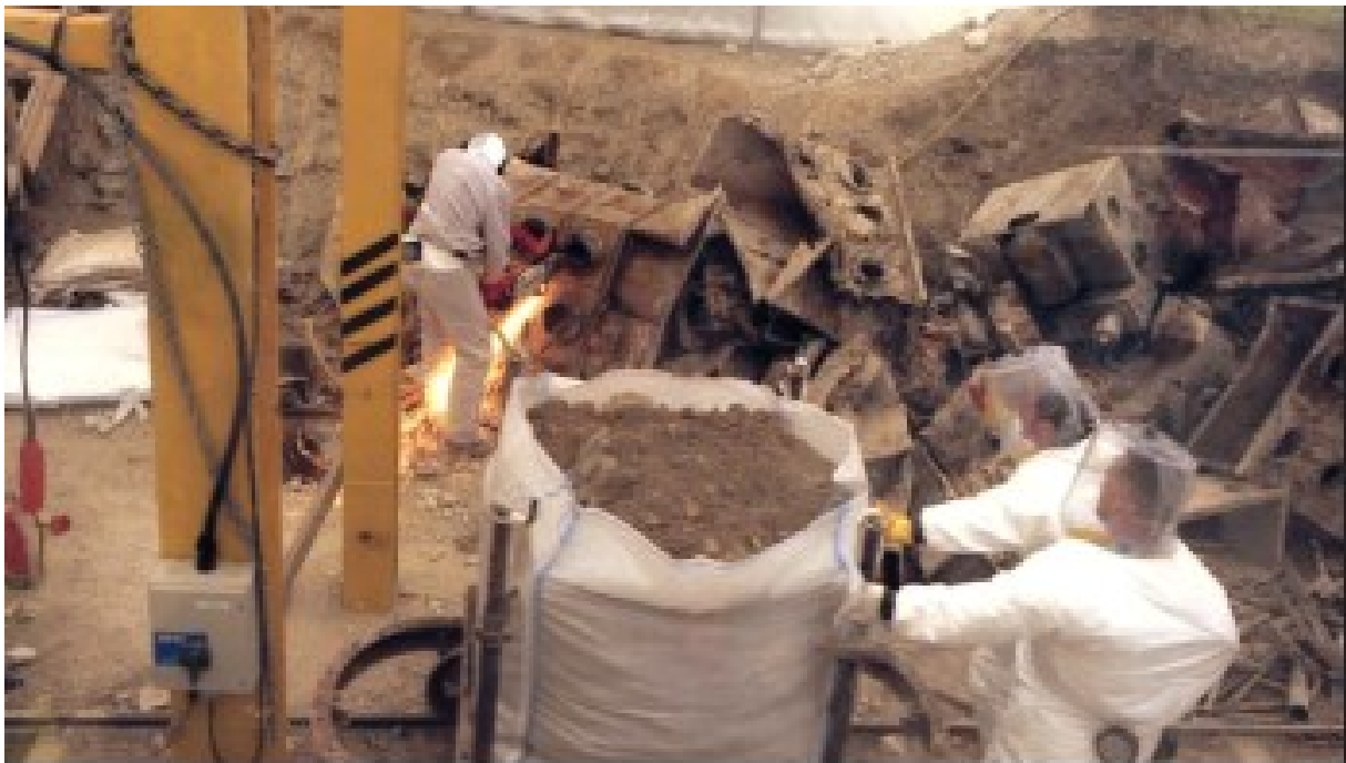
Clearing land contamination at Harwell
