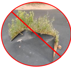
Failure to maintain liner
