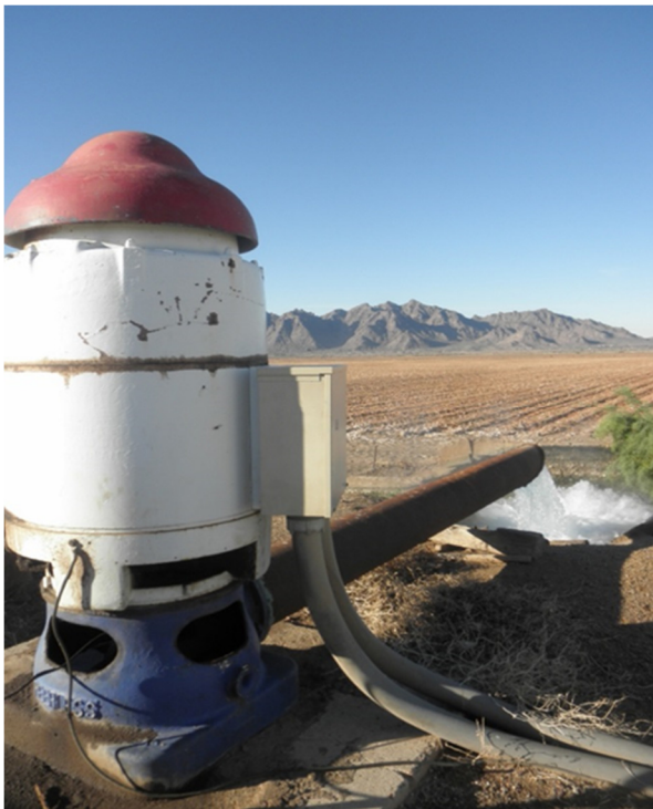
Figure 1 – Most groundwater pumped in Arizona is used for irrigation.
