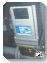
This photo shows an inverter panel of 6.6kW. The opening door is an optional item.
