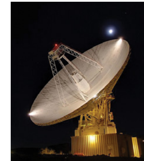
The 70-meter DSN antenna that houses the GSSR 450 kW transmitter.
