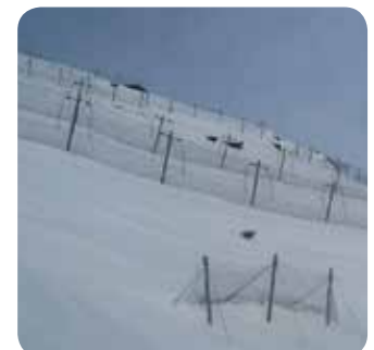
Dual protection wire net snow & rock fences
