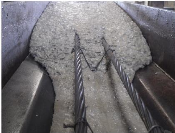
Fig. 2. Concrete pouring into the formwork.
