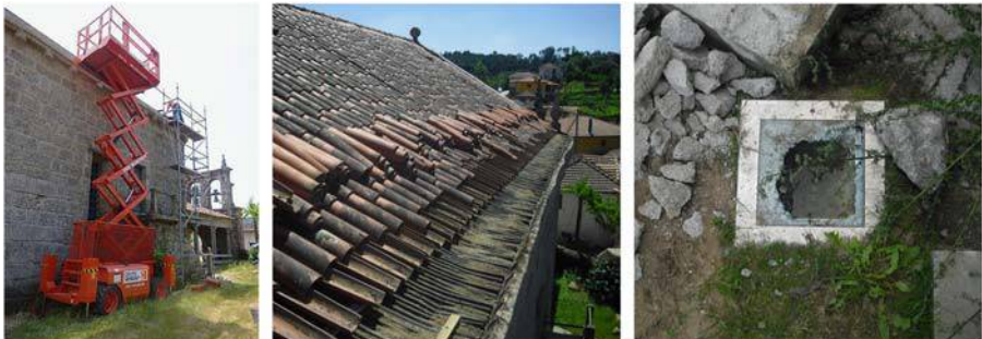
Plate 1. Maintenance works in pilot monuments, 2015
