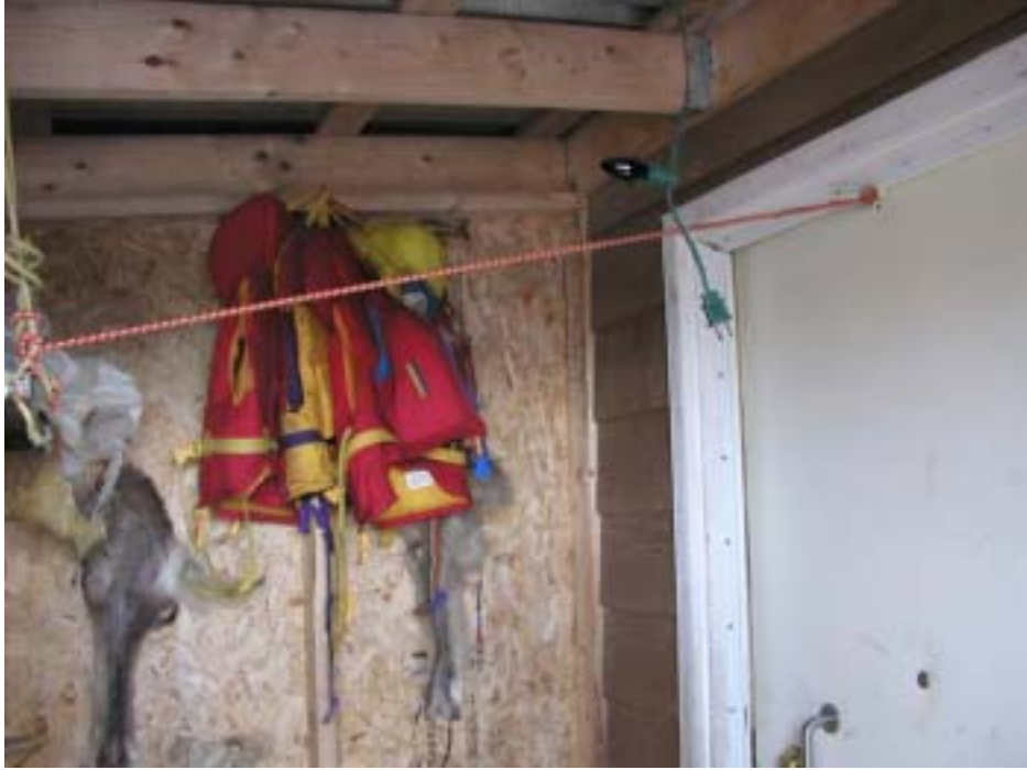
Figure 33. Bungee cords used to spring-load a house door so that it is not left open.
