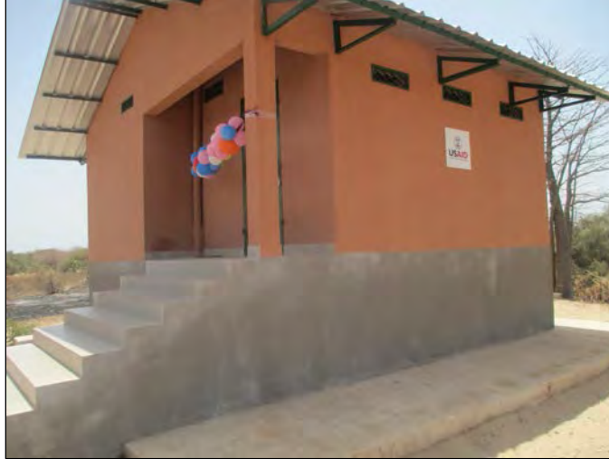
Figure 40. WASH toilet facility at the Kartong fish landing site
