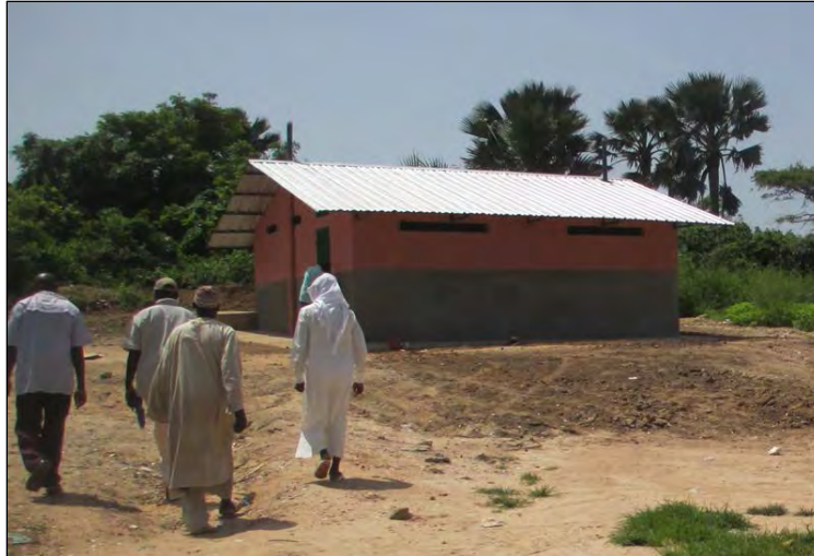
Figure 39. New WASH facilities at Brufut fisheries landing site.
