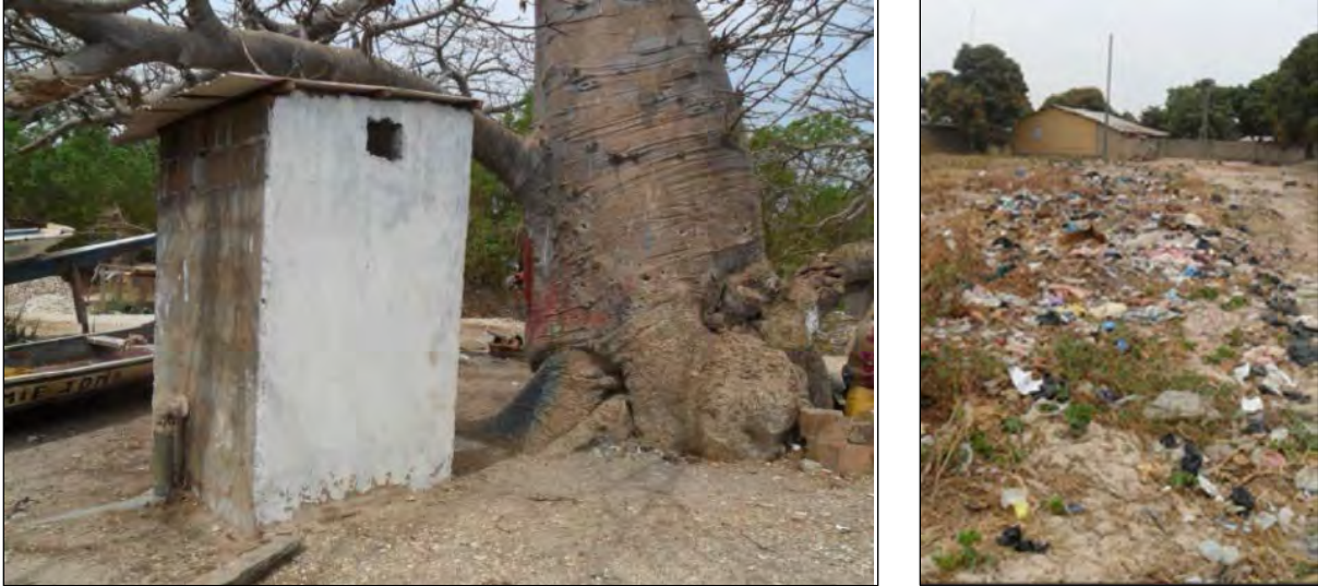
Figure 33. (from left) A latrine that emptied directly into the estuary and garbage disposal at oyster harvesting sites.
