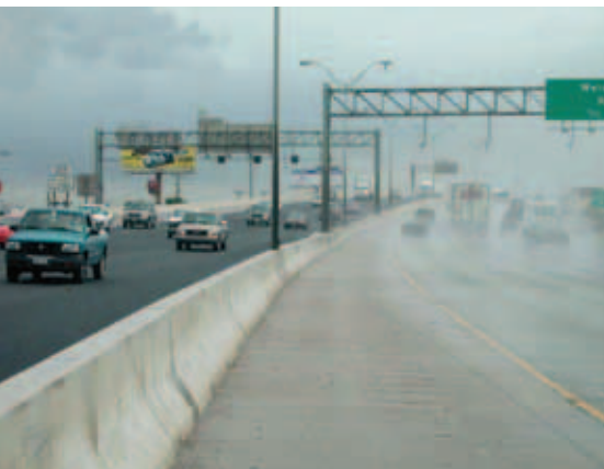
FIGURE 1 Visual comparison of the reduction in spray from PFC containing crumb rubber (left-hand lane) and continually reinforced concrete pavement (right-hand lane).
