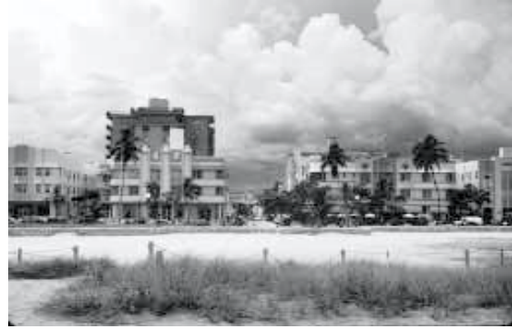
Courtesy of C. Galley
