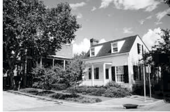
Courtesy of C. Galley
