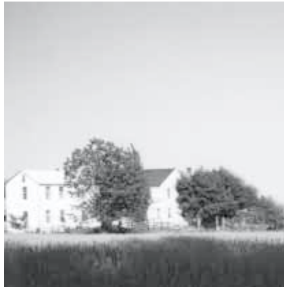
Courtesy of C. Galley
