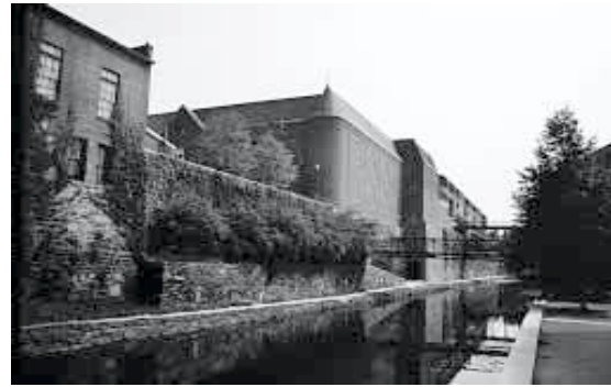
Courtesy of C. Galley
