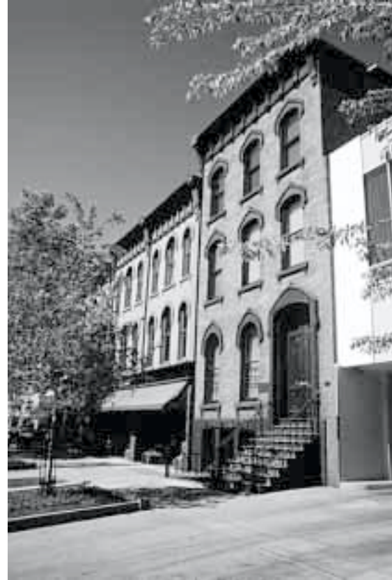
Courtesy of C. Galley
