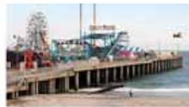
The Steel Pier Revitalization
