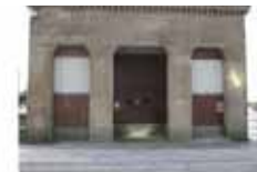
Clean and operable public restrooms
