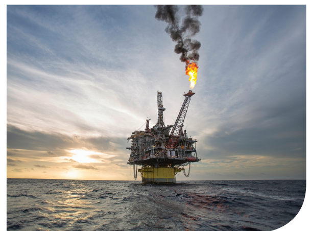
Natural gas platform in the Gulf of Mexico illustrates some of the infrastructure at risk from coastal storms.
