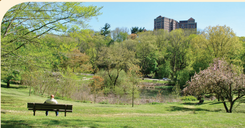
This one-acre stormwater wetland was constructed in Philadelphia to treat stormwater runoff in an effort to improve drinking water quality while minimizing the impacts of storm-related flows on natural ecosystems.
