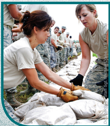
Members of the National Guard lay sandbags to protect against Missouri River flooding.
